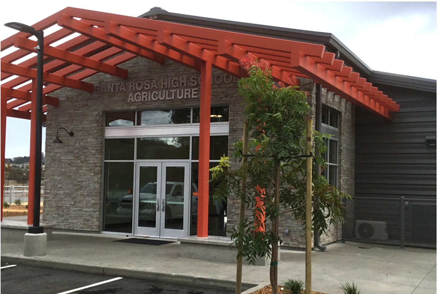
Santa Rosa High School Agricultural Facility (Arntz, PBK)
