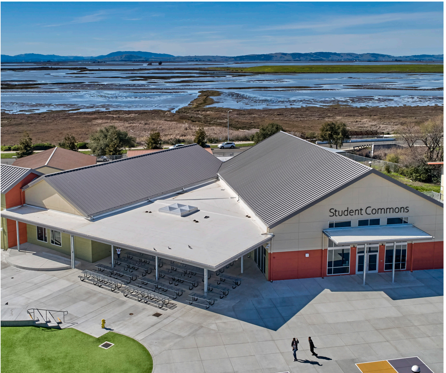
American Canyon Middle School Design Build (Arntz, PBK)
