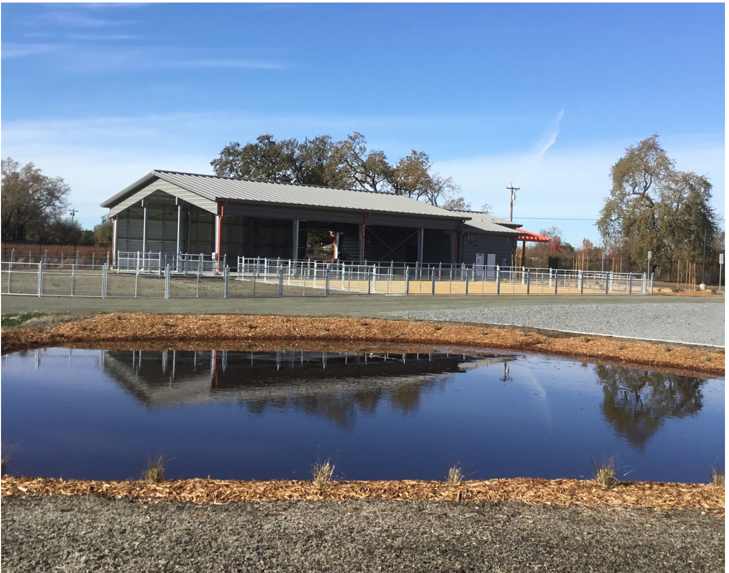
Santa Rosa High School Agricultural Facility (Arntz, PBK)
