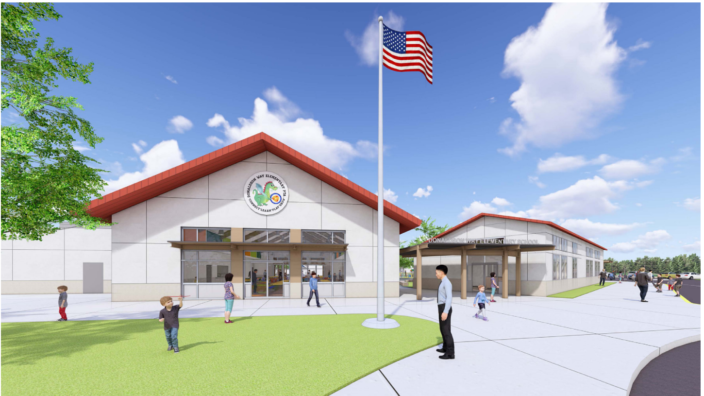
Donaldson Way Elementary School Design Build (Arntz, PBK)
