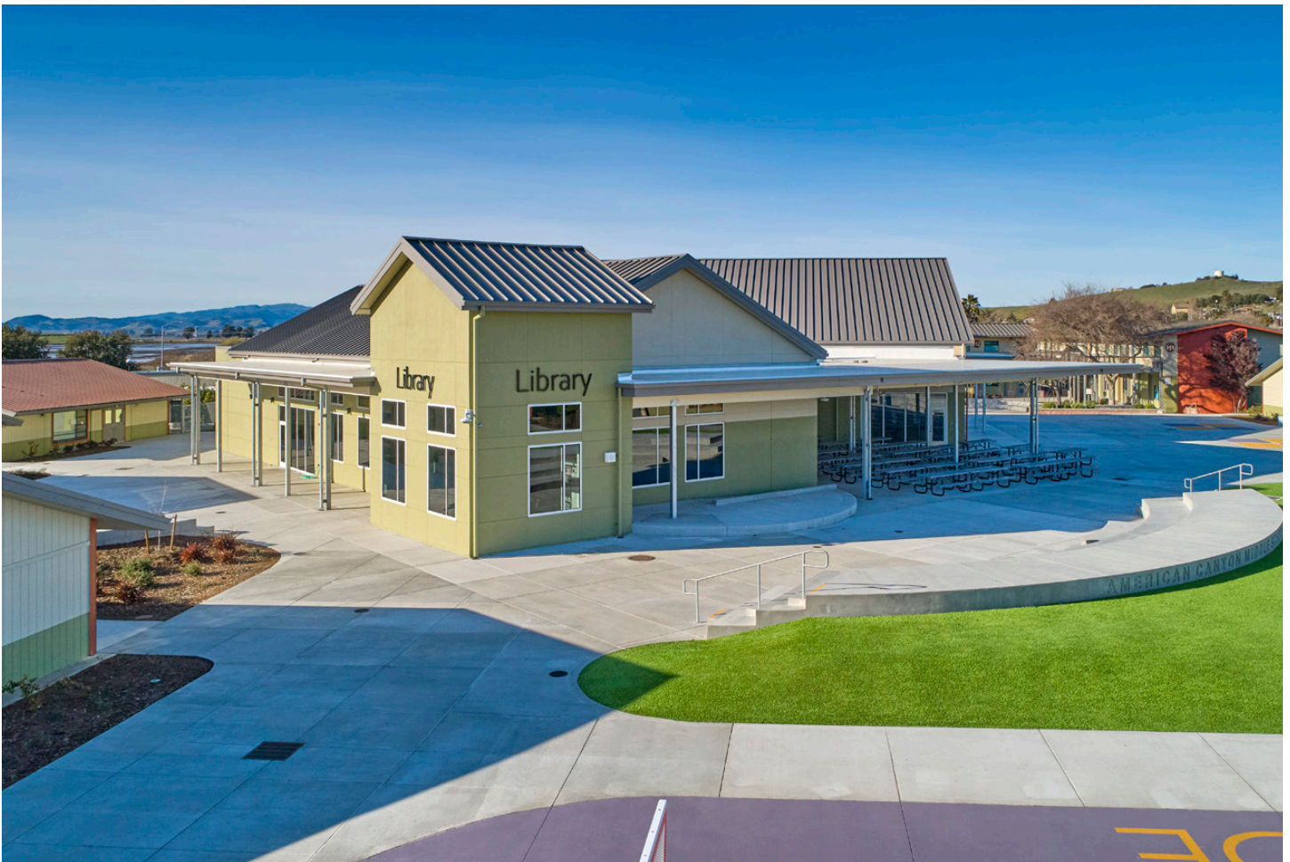
American Canyon Middle School Design Build (Arntz, PBK)
