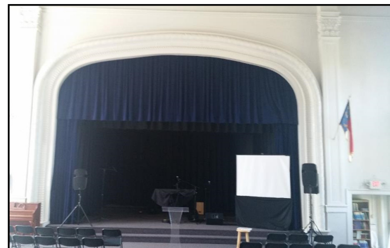
Proscenium surround detail at stage
