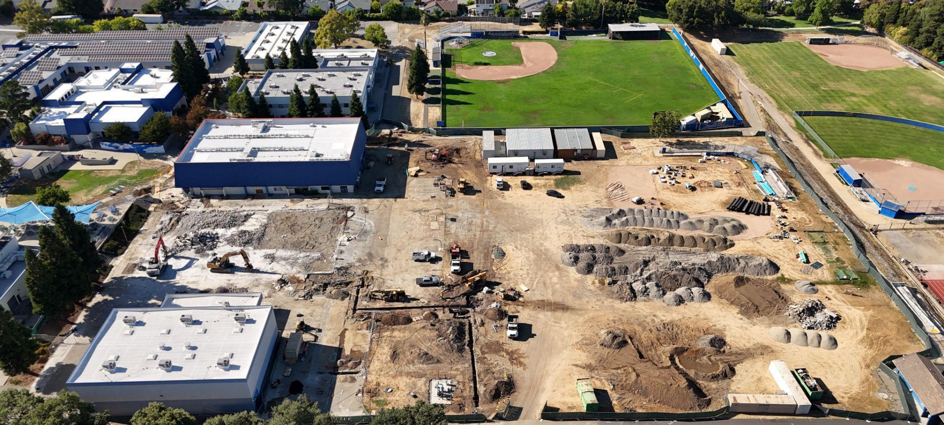
Foothill HS - Construction Site
