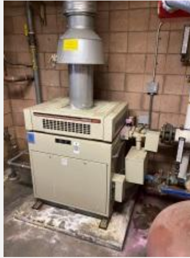
(E) BOILER SYSTEM to be demolished
