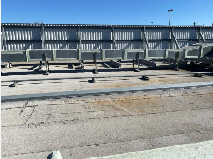
(E) ROOFING SYSTEM CONDITION to be removed and replaced
