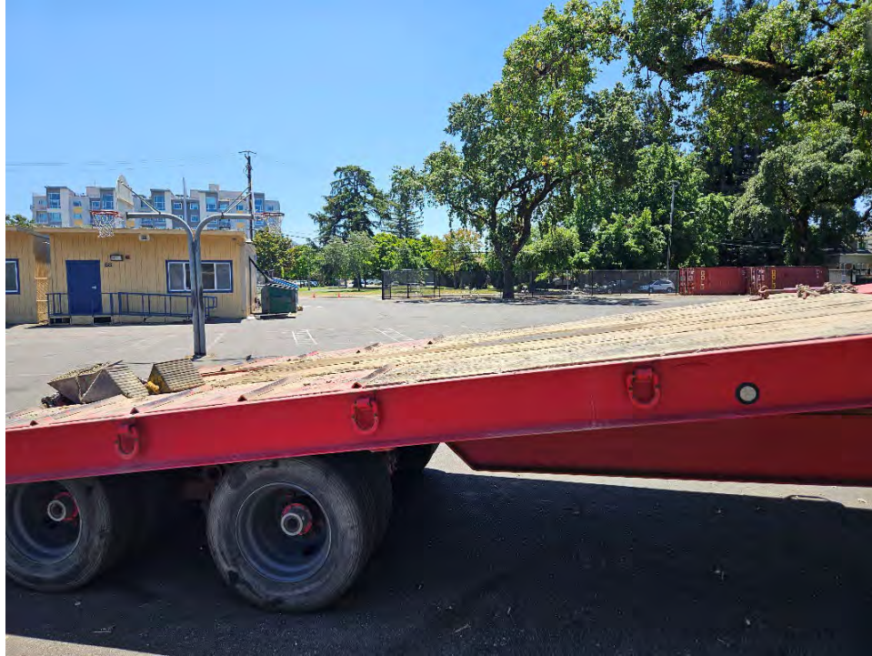
Photo 3: Site overview. View of proposed site of Zinnia Building E, facing southeast towards 5 th Street.
