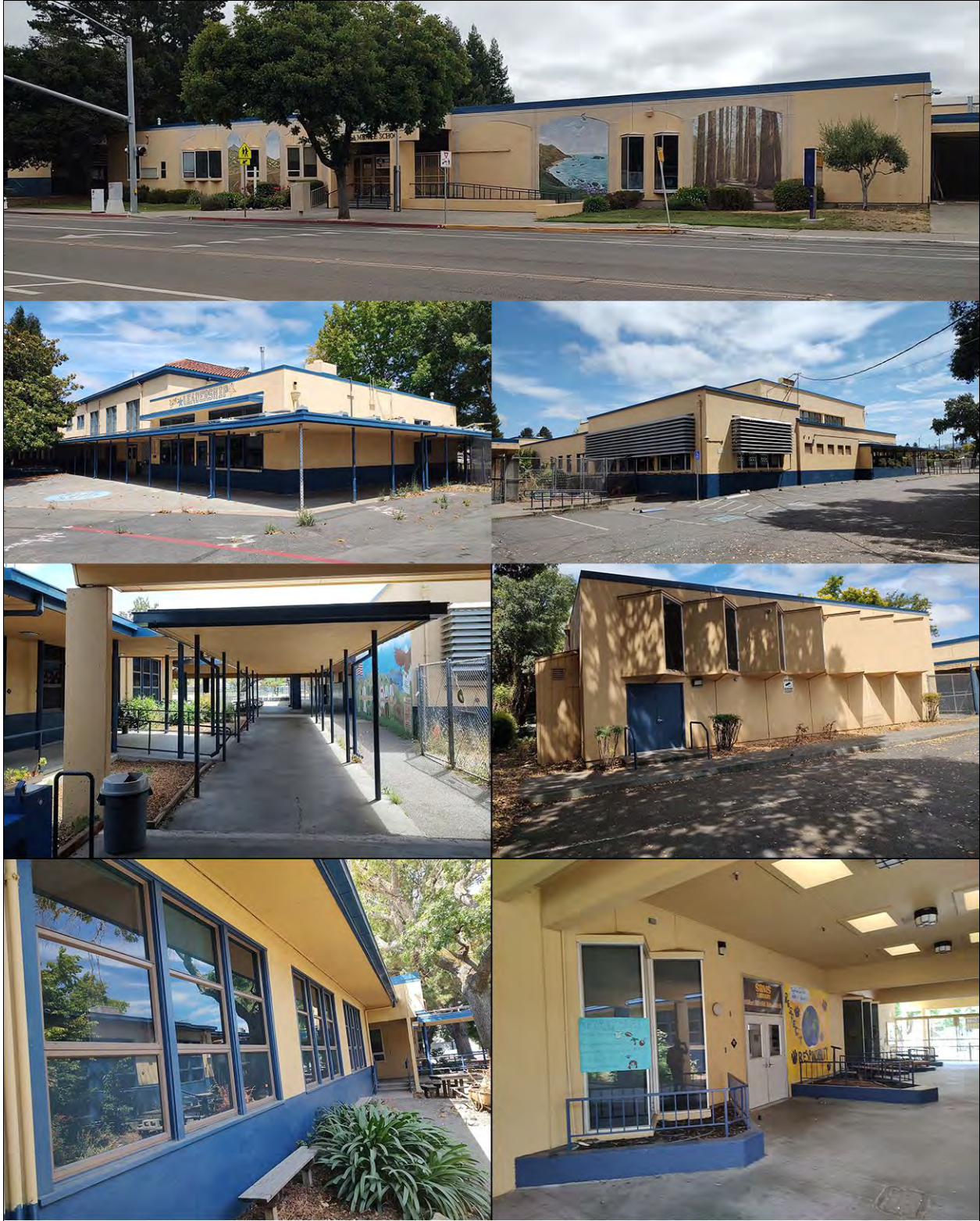
Figure 8. Typical buildings at Santa Rosa Middle School. Clockwise from the top : frontage along E Street; gym and weight room; art building; library entrance; typical classroom windows; covered walkways; leadership center, cafeteria and Cougar's Den. (Photographs taken on July 23, 2025)
