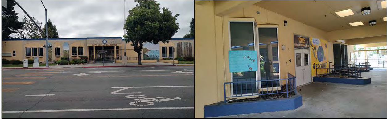
1970-1971 additions. Left : main entrance fronting E Street, view to the east; right : library entrance, view to the southwest
