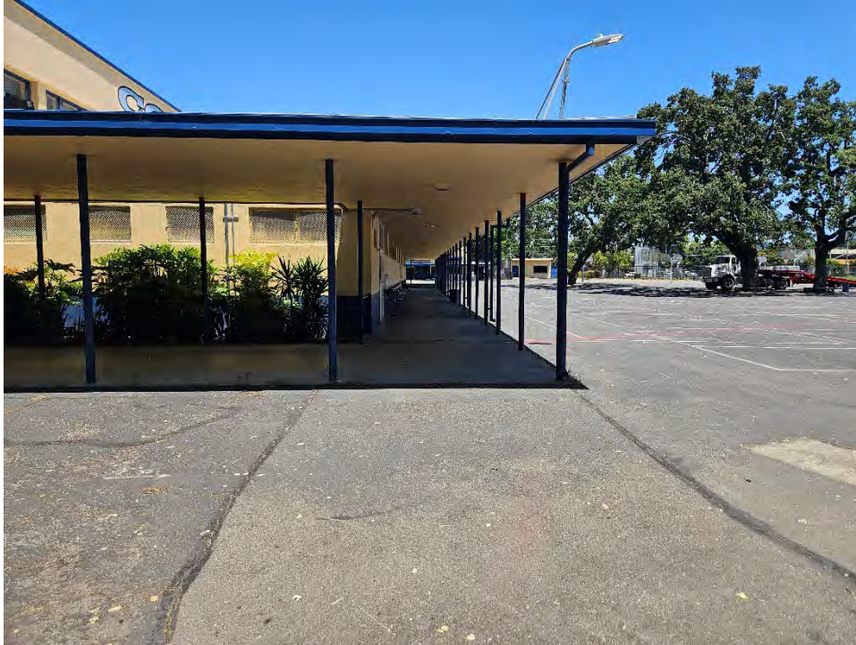
Photo 11: Site overview. View of the gymnasium and pavement adjacent to proposed construction, facing north towards College Avenue.
