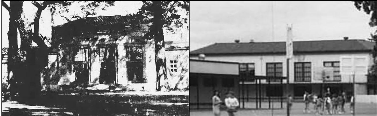
1939 auditorium. Left : ca. 1939, view to the east (source: Santa Rosa Republican 1939a); right : ca. 1958, view to the northwest (source: Santa Rosa Junior High School 1958 Yearbook)
