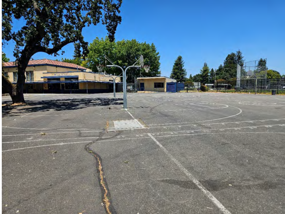
Photo 1: Site overview. View of Building F and Building L, facing northwest towards the intersection of College Avenue and E Street.
