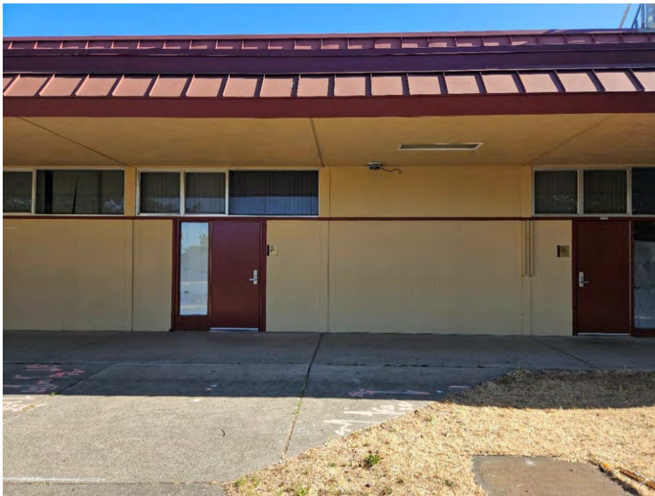
Photo 10: Site overview. View of Building B, to the north of location of proposed Folia Building.
