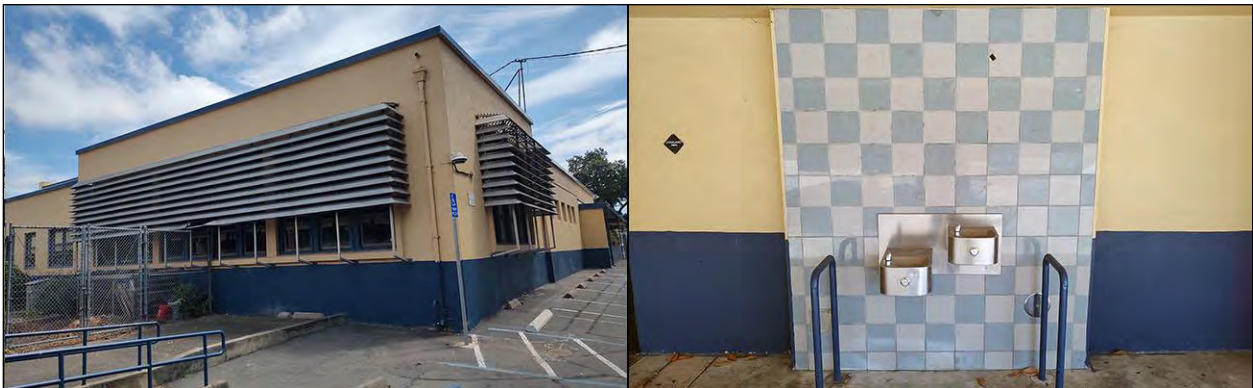
1950s additions. Left : gymnasium, current weight room, view to the northeast; right : tile wall backing water fountain on cafeteria from 1950 remodel
