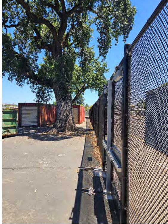
Photo 9: Site overview. View of fence along southern boundary of campus, facing east.
