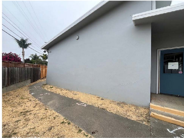
Location 1 - View to northeast of low northeast-facing scarp at northern corner of main building, approximately coincident with fault trace mapped by Hecker (2016, 2018) and CGS (2024). Note approximate 1-foot rise in ground surface against block wall and prominent cracks in stucco facade.
