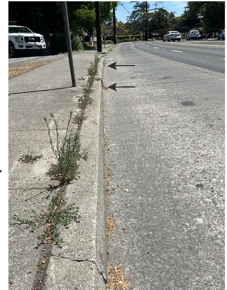
Photo 5 - View to northeast of right-lateral offsets between sidewalk panels along Fourth Street. Total of 4 locations noted with apparent cumulative offset just under 3 inches.
