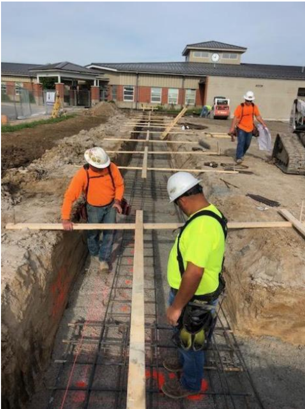
South concrete footing rebar install – Gymnasium
