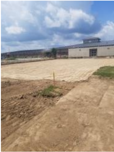
Photo 1 Gymnasium Subgrade below LVC - Overall
