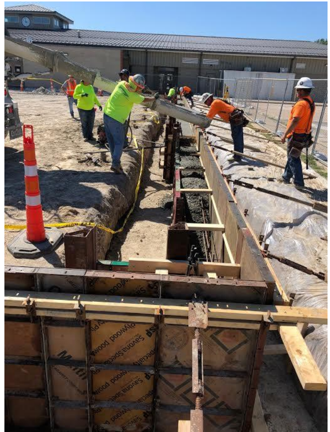
North concrete foundations and piers being placed – Gymnasium
