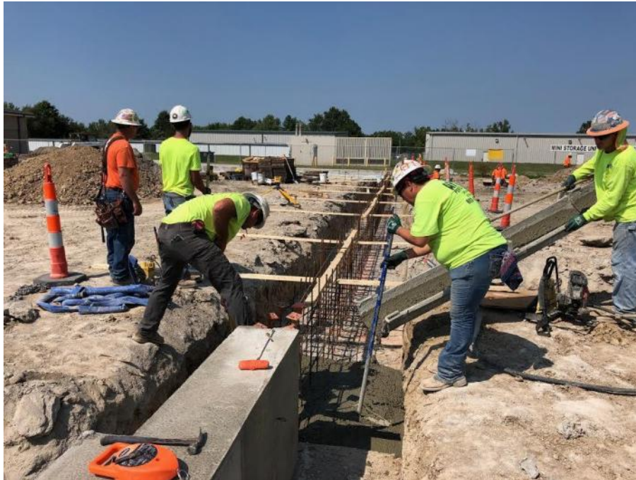
East concrete foundation being placed – Gymnasium
