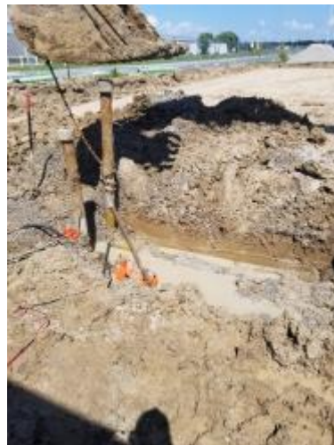
Photo 6 Pipe removal at approximately 6' down from Slab on grade/ Ponding Location #2
