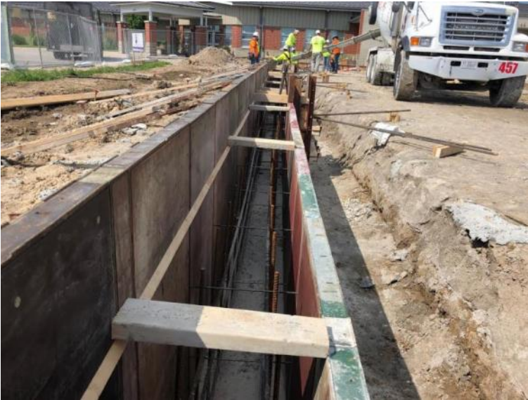
South concrete foundations and piers being placed – Gymnasium
