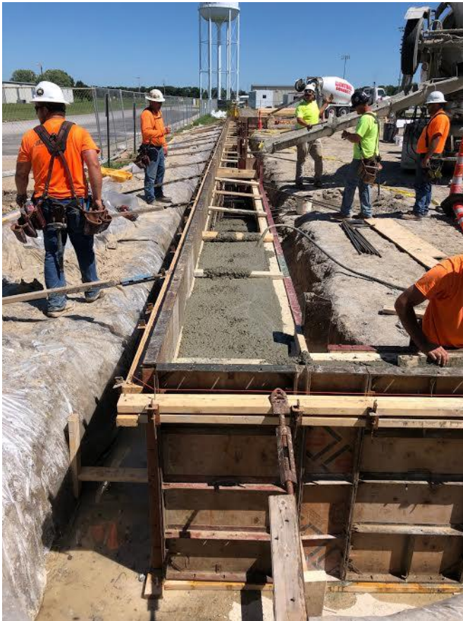
North concrete foundations and piers being placed – Gymnasium
