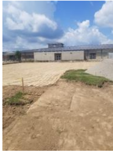
Photo 2 Gymnasium Subgrade below LVC - Overall
