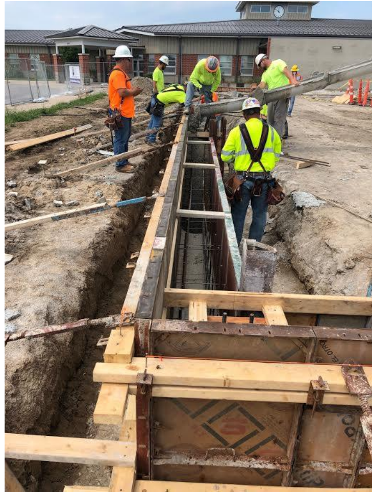
South concrete foundations and piers being placed – Gymnasium
