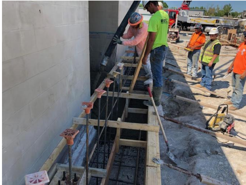
West concrete foundations being placed – Gymnasium
