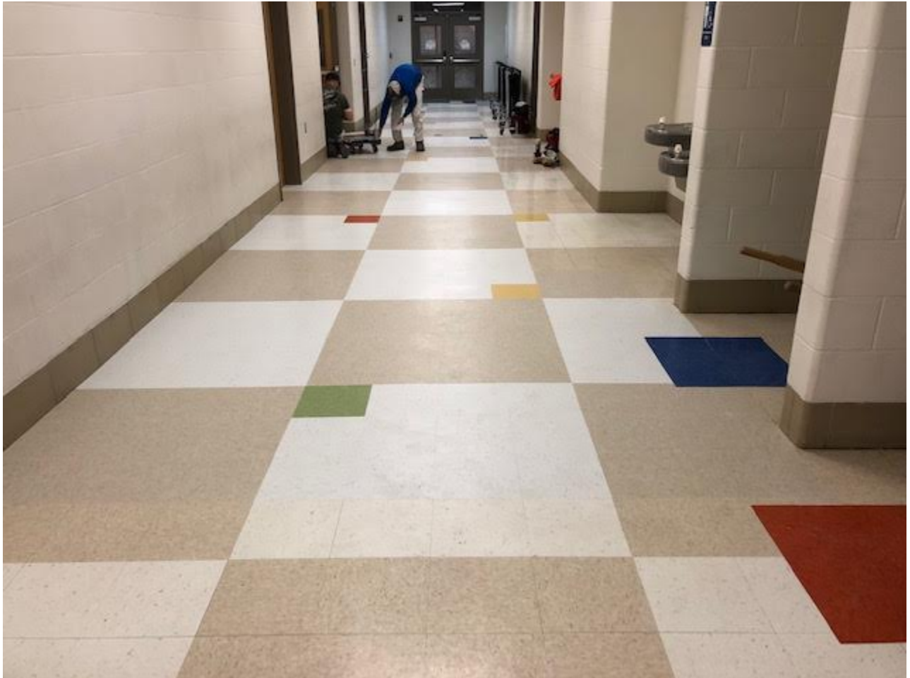
Existing School Corridor – New Sanitary Line Flooring Installed
