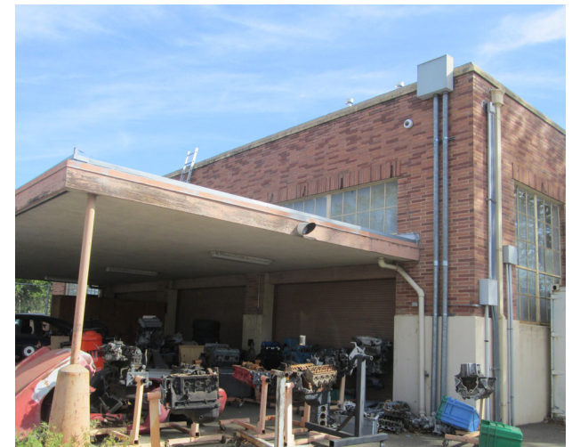
Shop Building Exterior
