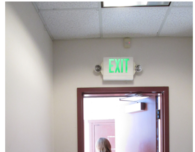
North Gymnasium Interior
