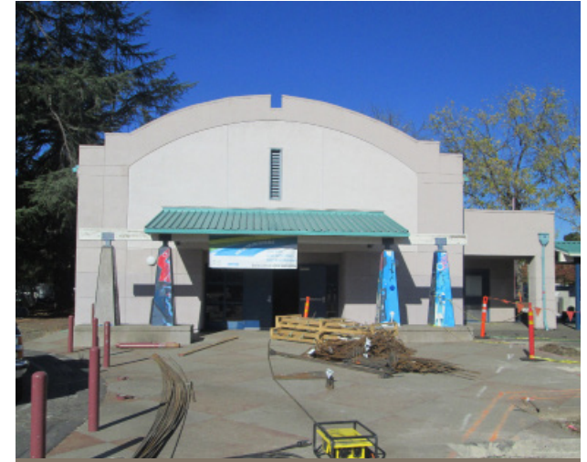
Multi-Purpose Building Exterior
