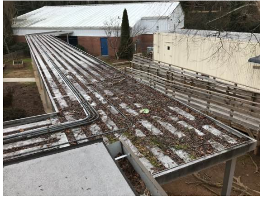
Clean Aluminum Covered Walkway/Gutters
