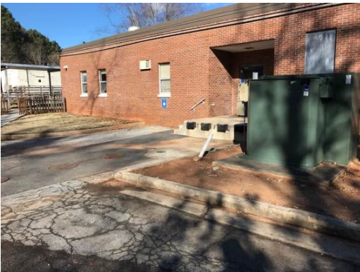
Replace Bollard And Asphalt At Kitchen Loading Dock
