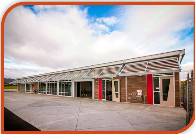
Gen7 STEAM Modular Classrooms—open to the outside
