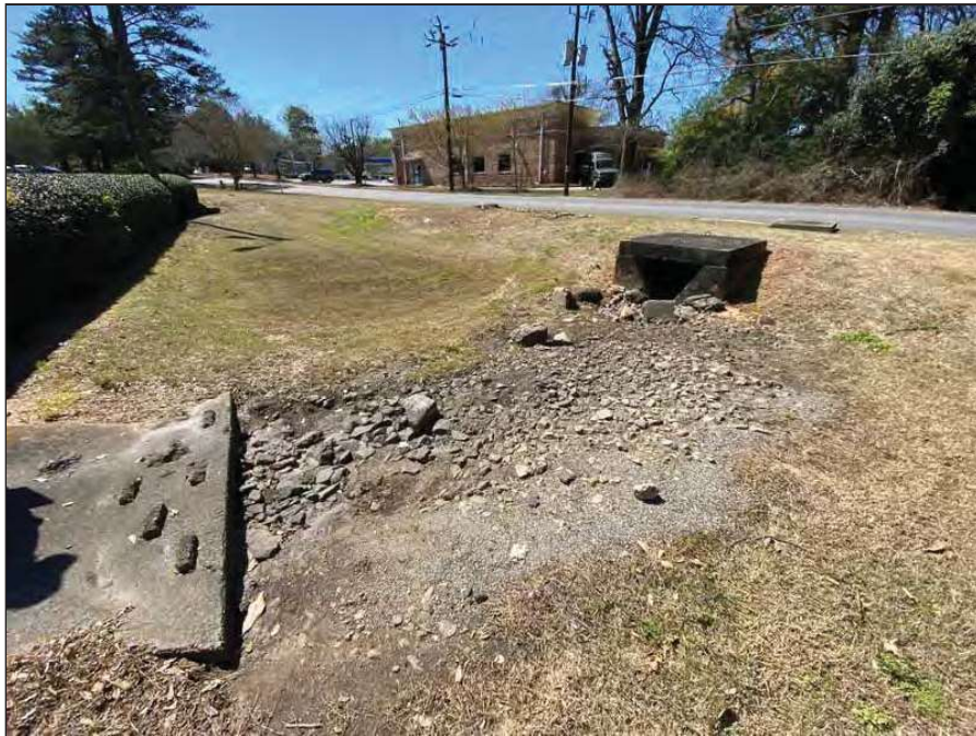
62 - Culvert on the western property boundary
