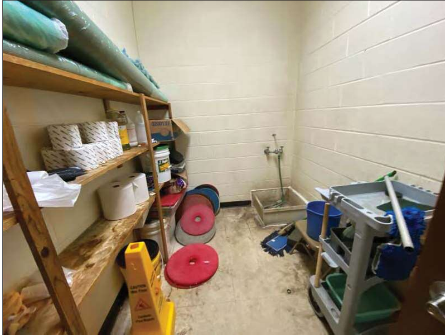
45 - Janitors closet on the first floor
