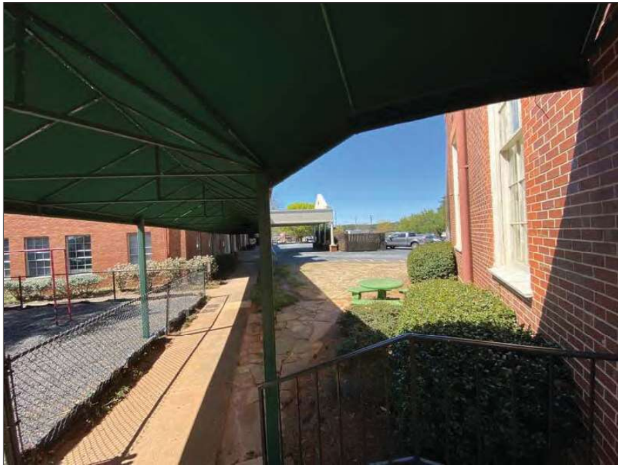
10 - Southern view of Mulligan Hall
