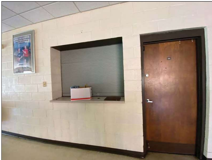
42 - Concession stand on the first floor
