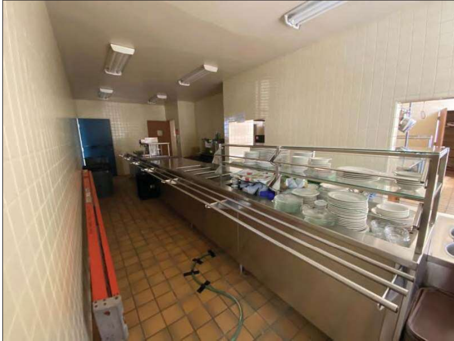
15 - Kitchen on the first floor
