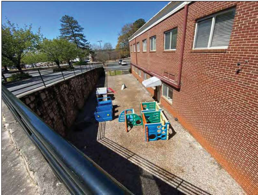
34 - Playground on the northern side of the Family Life Center
