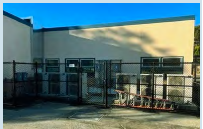
Sun Valley HVAC upgrades
