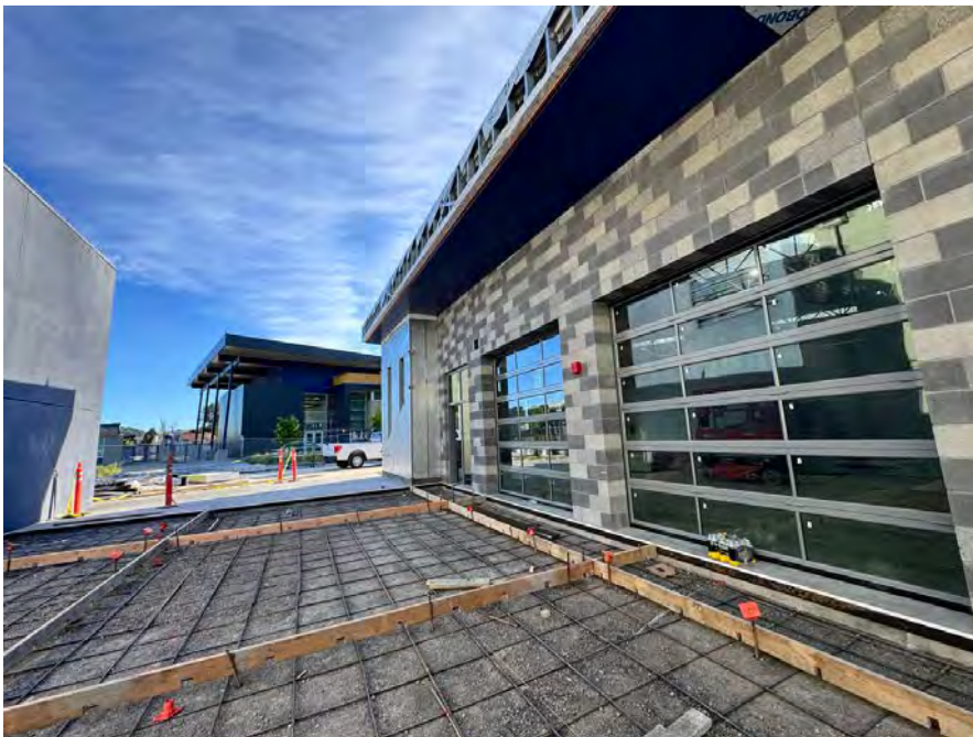
Terra Linda High School aquatic center construction
