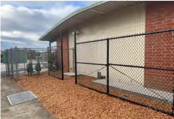
Glenwood Elementary HVAC installation
