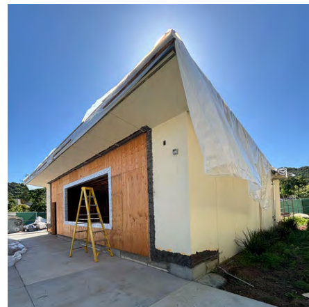
Venetia Valley buildings G and H modernization
