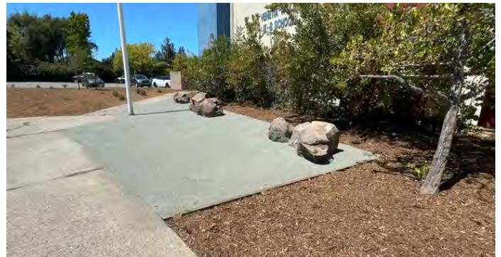
Venetia Valley landscape improvements
