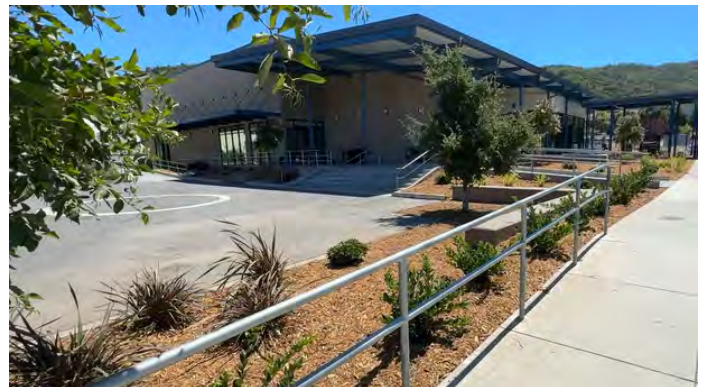
Venetia Valley landscape improvements
