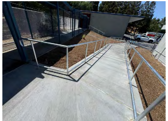
District Office Annex new ADA ramp and access
