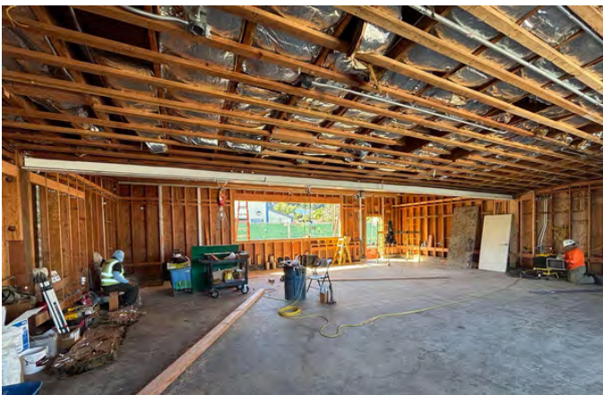
Venetia Valley buildings G and H modernization
