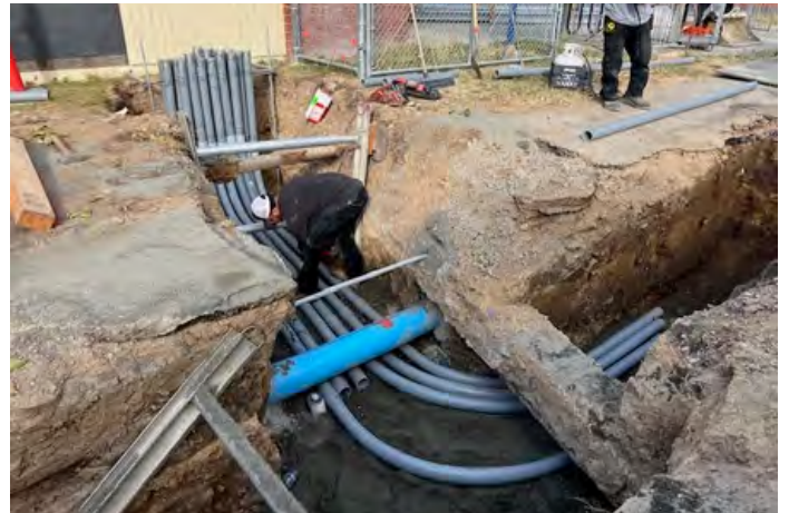
Glenwood Elementary underground conduit work
