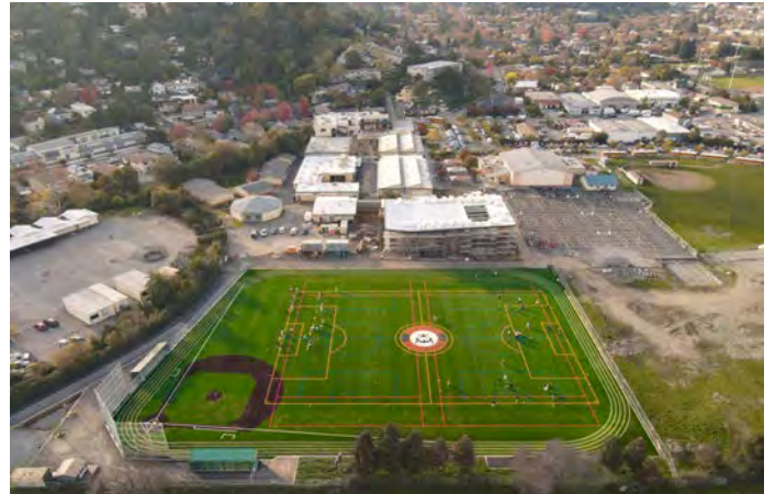
Davidson Middle School aerial view of fields
