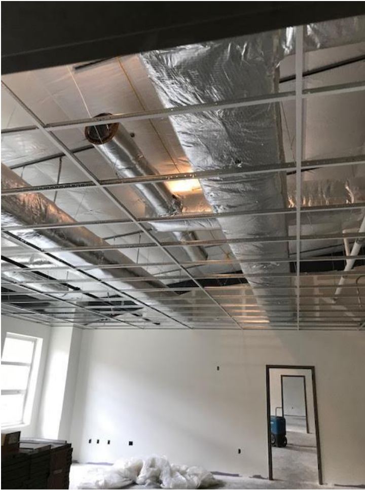
Classroom – Ceiling Grid
