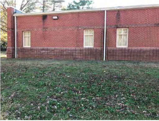
Power Wash Exterior
