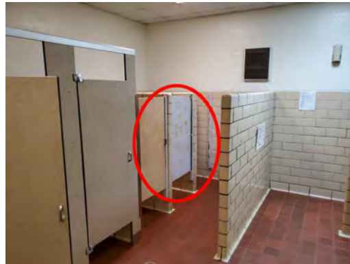
Add New Toilet Partition
