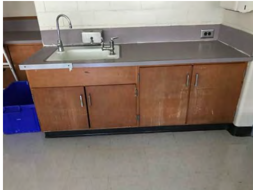
Refinish Lower Cabinets In K And Pre-K Classrooms
