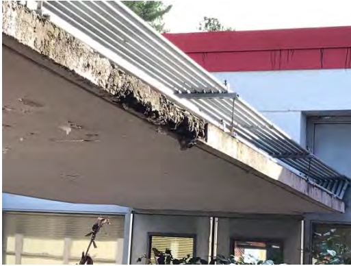
Repair Concrete Awning Over Sidewalk Between School Wings At Interior Courtyard
