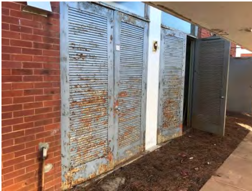
Paint Exterior Doors To Mechanical Room
