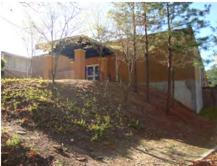
24-Mar-2011 North Elevation
