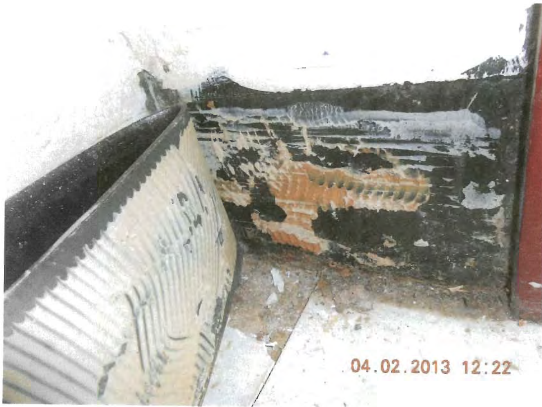
Photo #4 – Cove base mastic – dark tan
