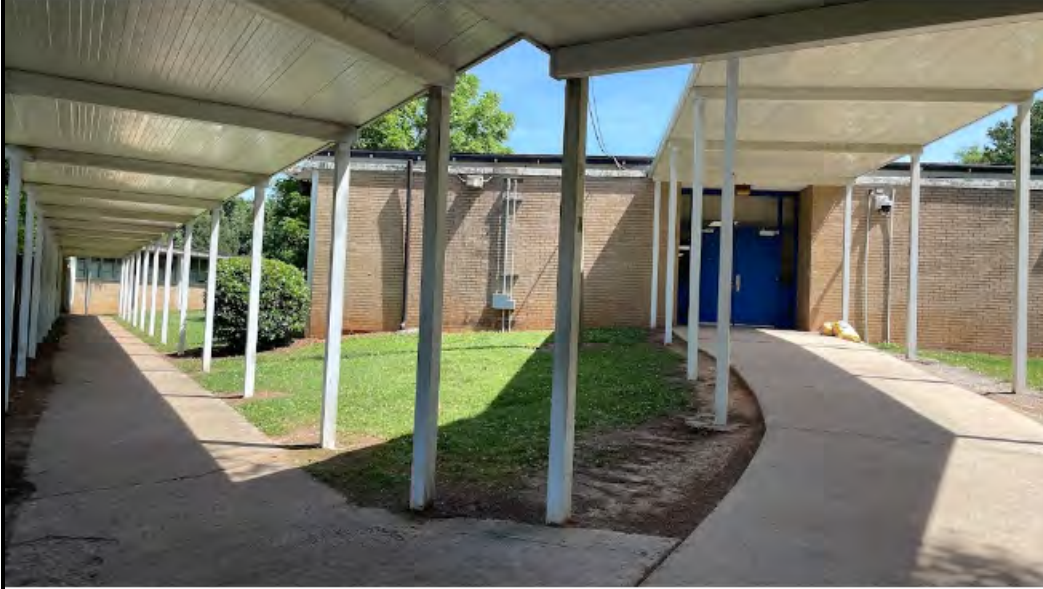
Picture 13: Covered sidewalk between the school building and the gymnasium building.
