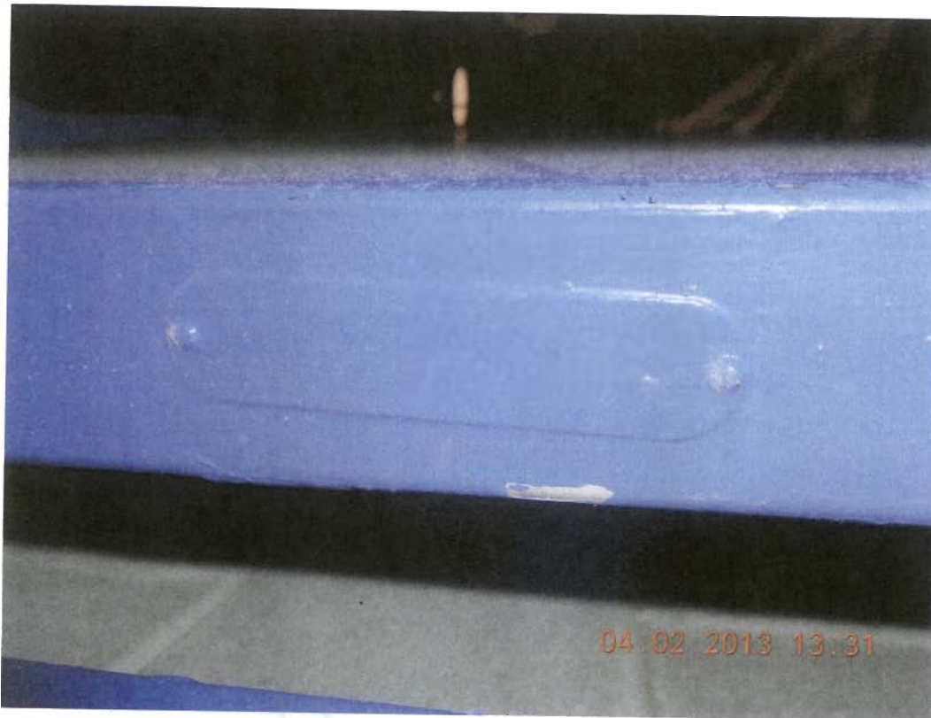
Photo #5 – Fire doors – PACM*
