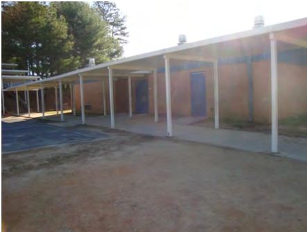
24-Mar-2011 North Elevation
