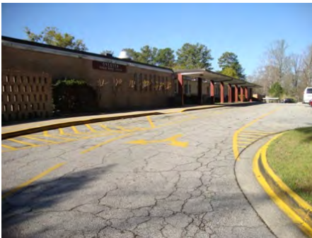
24-Mar-2011 North Elevation
