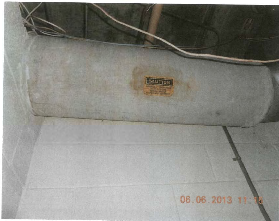
Photo #10 – Hot water heater flue – PACM*
