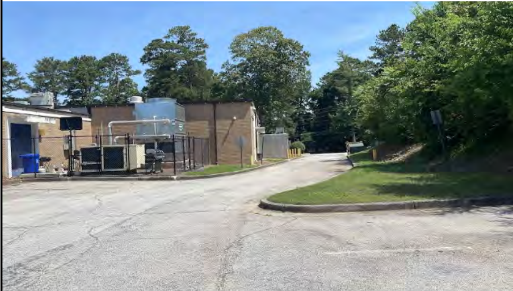
Picture 16: East driveway and scool building.
