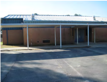
24-Mar-2011 North Elevation
