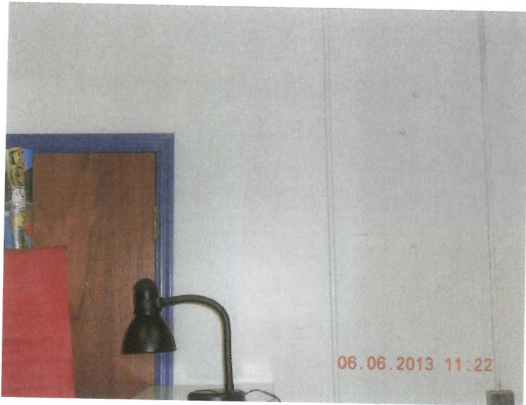
Photo #13 – Wallboard and Joint compound
