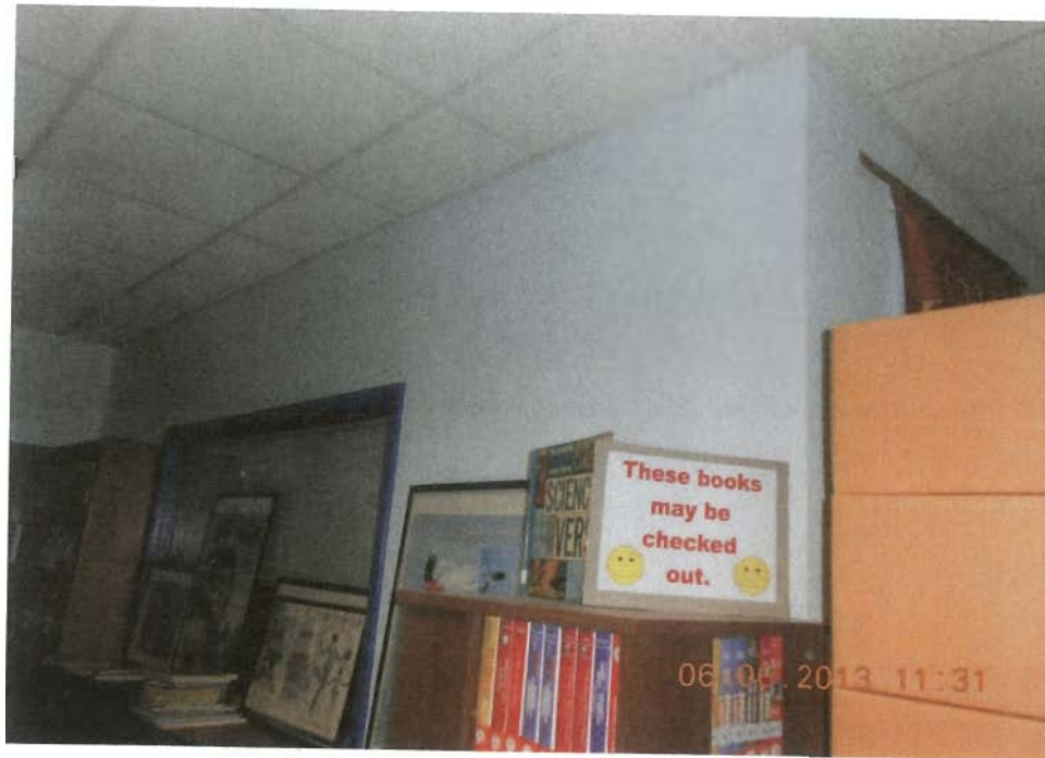
Photo #1 – Wallboard and joint compound
