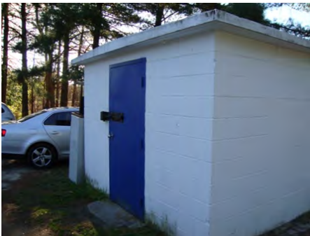
24-Mar-2011 North Elevation
