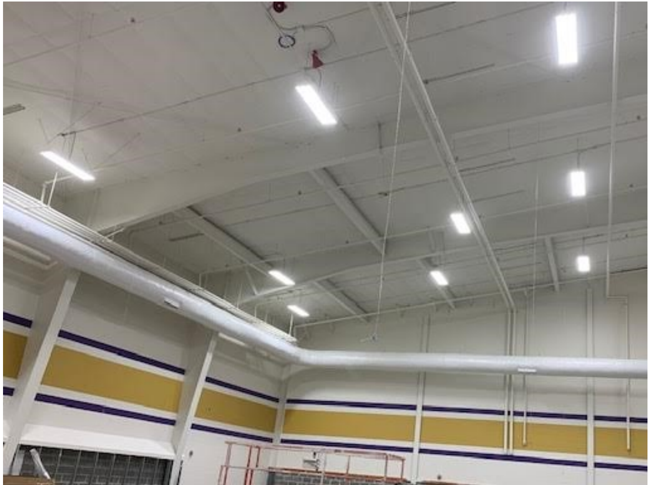
Gymnasium – Interior View
