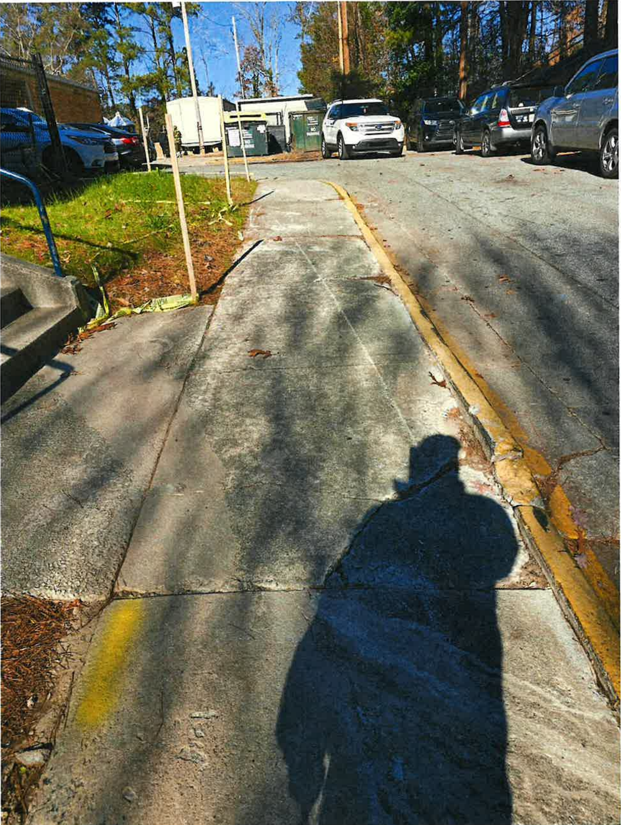
Henderson Mill Existing 1
