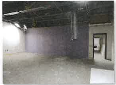
Replacement of operable partitions.
