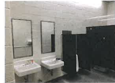
Complete replacement of restrooms
