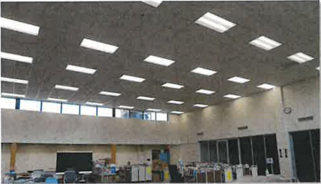
Ceiling & lighting replacement
