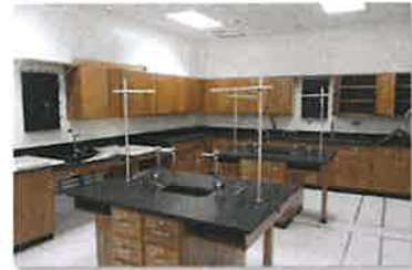
Science Lab renovations
