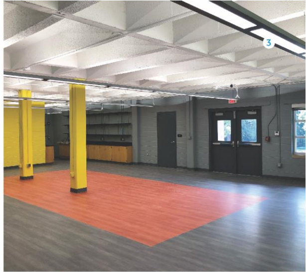
1. Rendering of Interior Renovation 2. View of interior renovation at substantial completion
