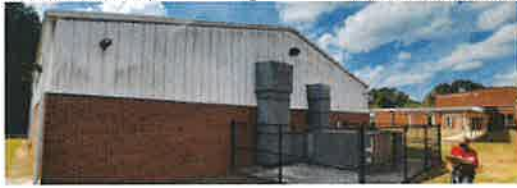
Pine Ridge Elementary School
