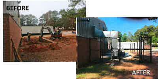
Above: New HVAC for Gymnasium, Below: ADA Bathroom upgrades
