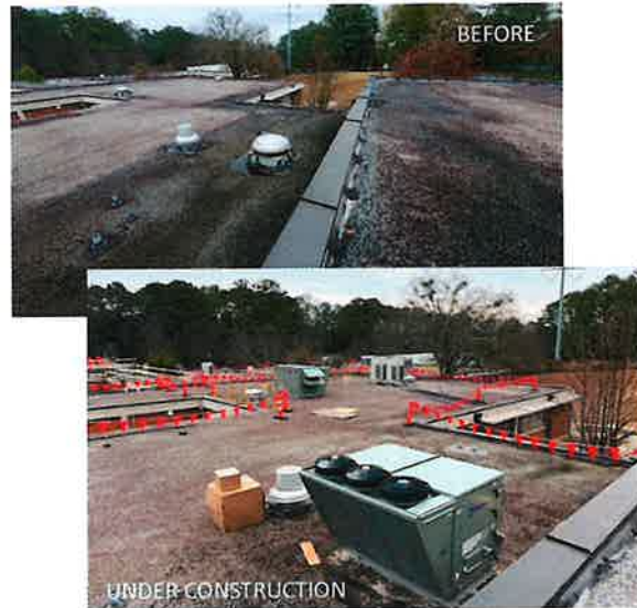
Above: New RTU's, OAU's, and VRV's set on roof.
