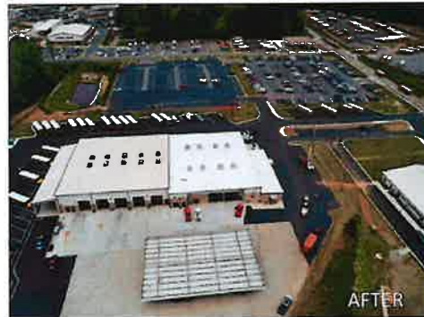
Phase 4: Bus Shop Addition and Renovation. Fuel Island canopy updated
