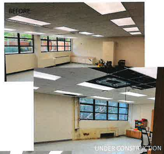
Middle: Unit Ventilators being removed and VRV's set in ceiling.
