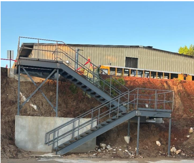
New stairs at Sam Moss
