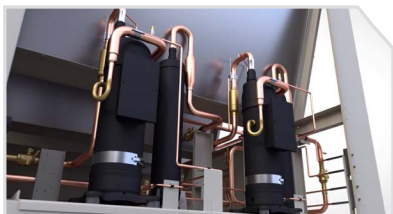
Inverter Scroll Compressors
