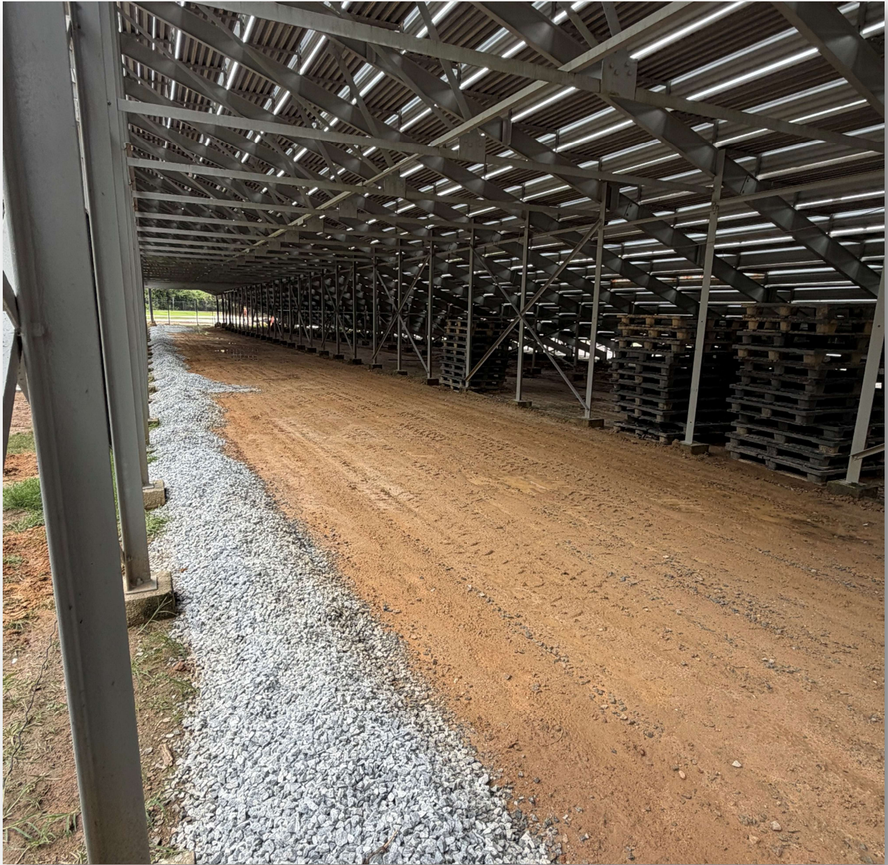
57 stone installation under WBHS home bleachers on-going
