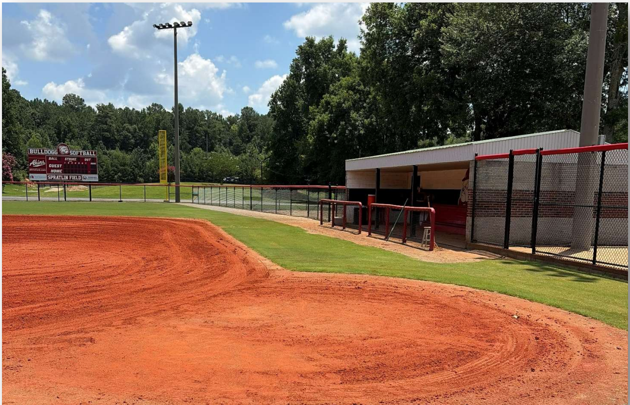
New fencing & top cap installed at WBHS softball field
