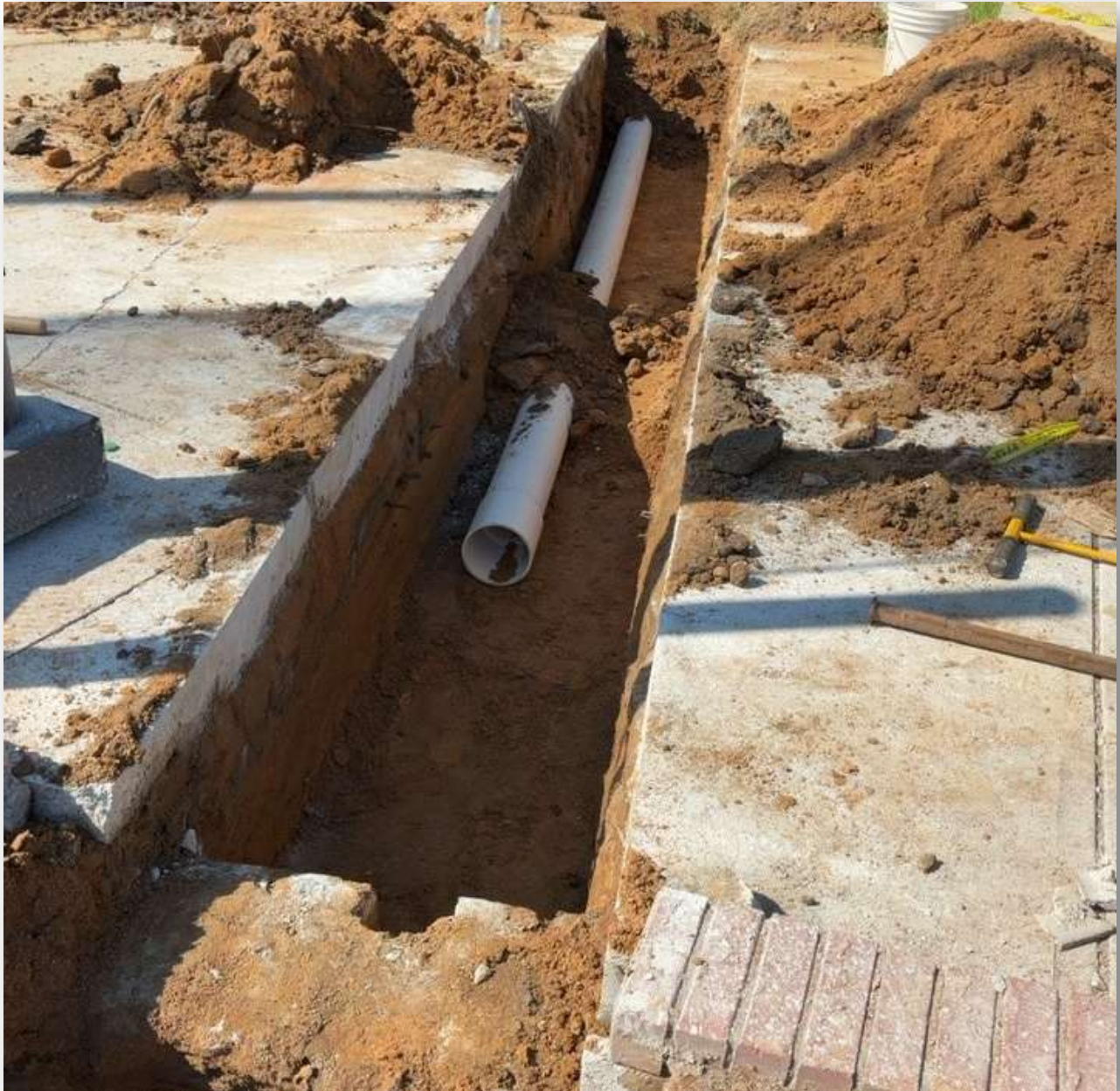
WBHS baseball maintenance drain installation on-going
