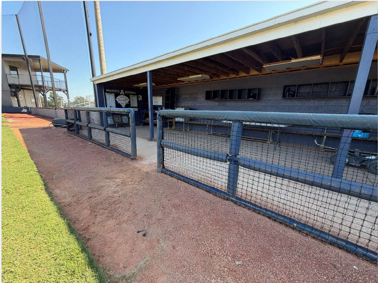
New dugout netting installed at Apalachee HS baseball field
