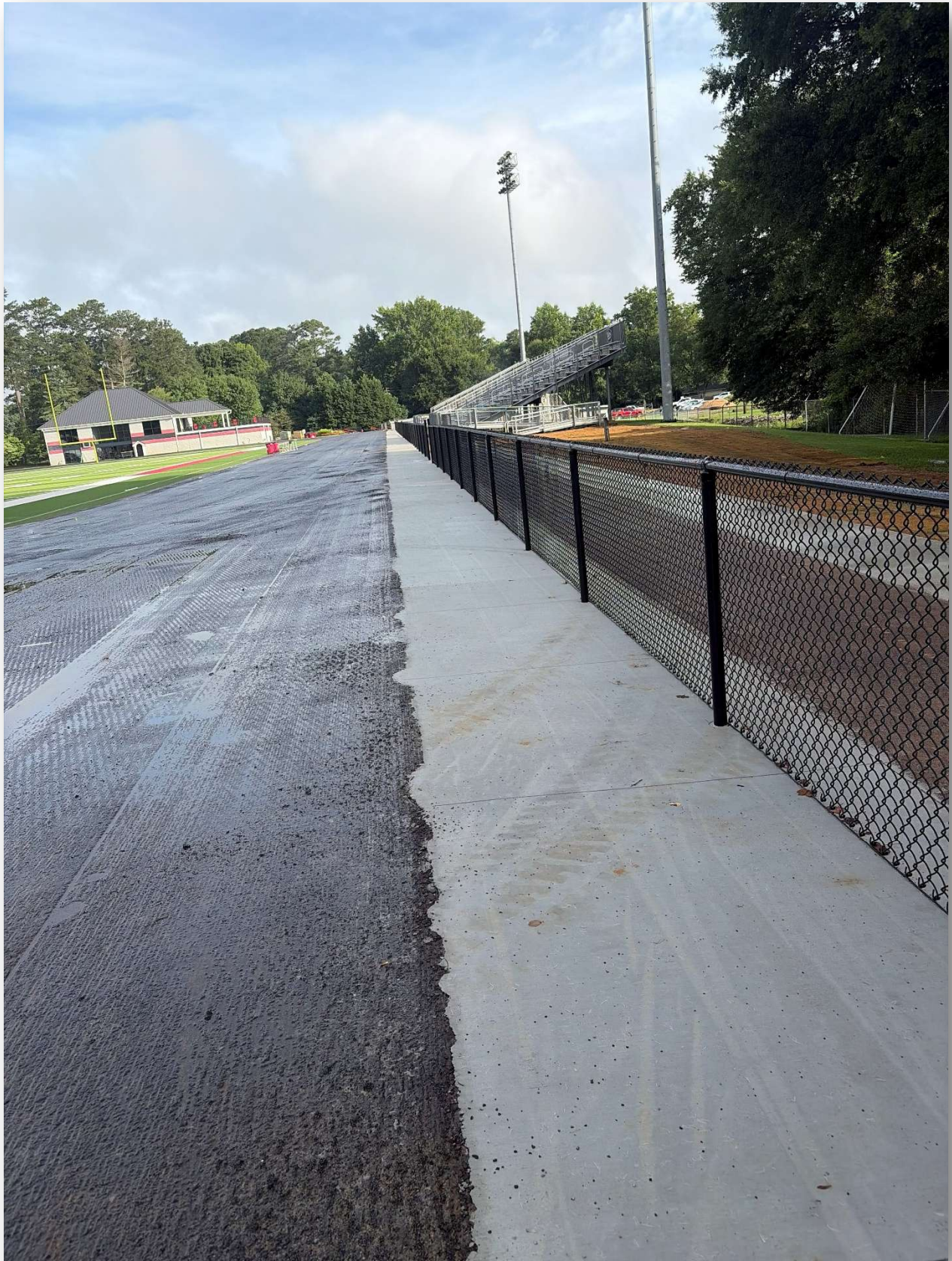
New track perimeter concrete & fencing at Winder-Barrow HS
