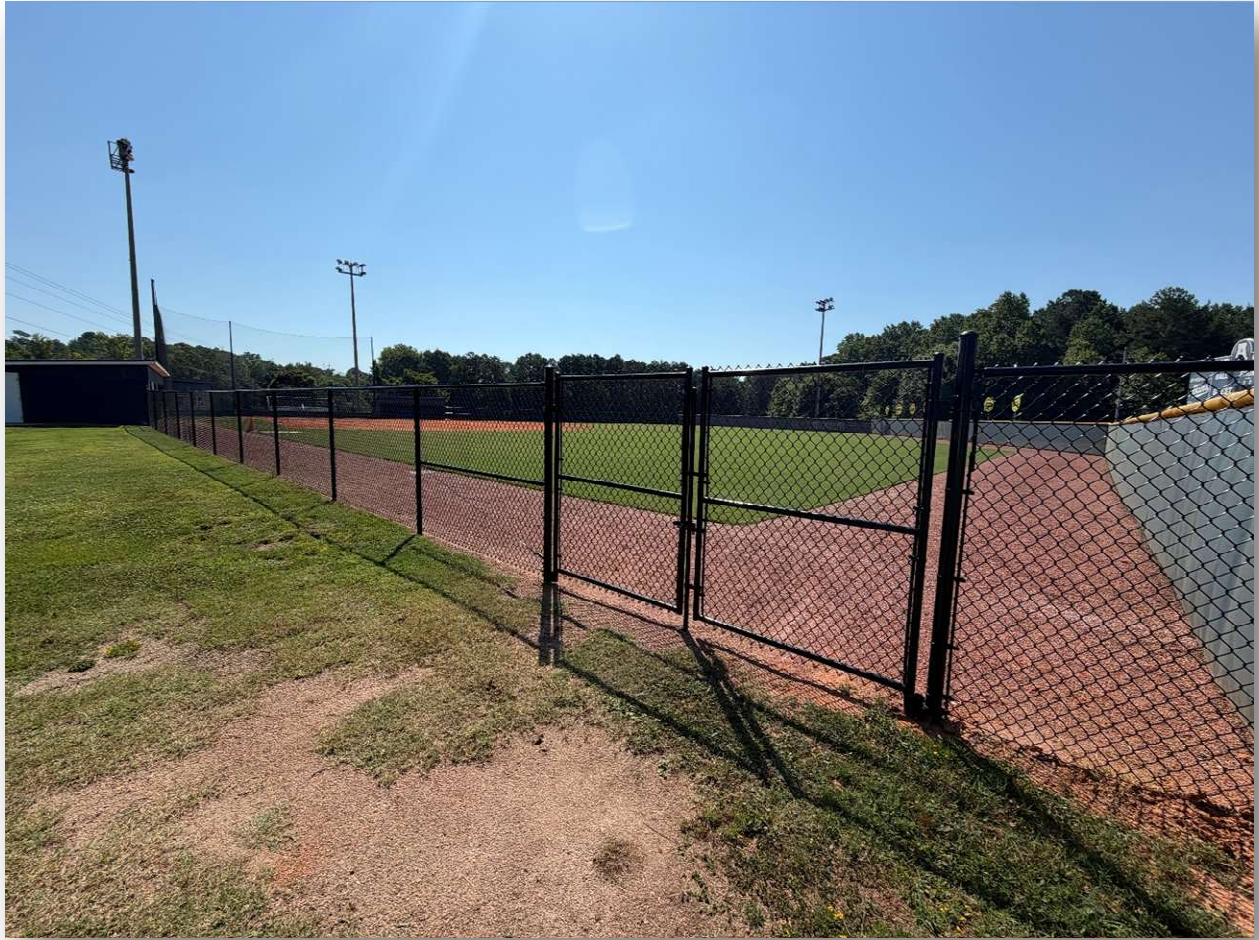
New fencing & gates installed at Apalachee HS softball field
