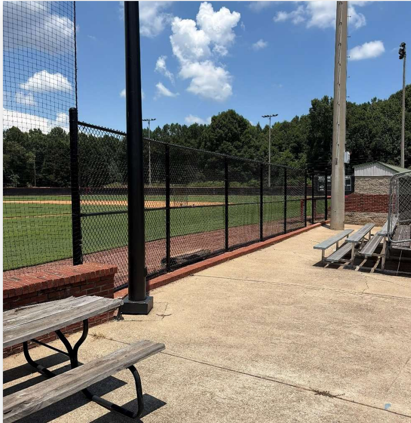
New fencing installed at WBHS baseball field
