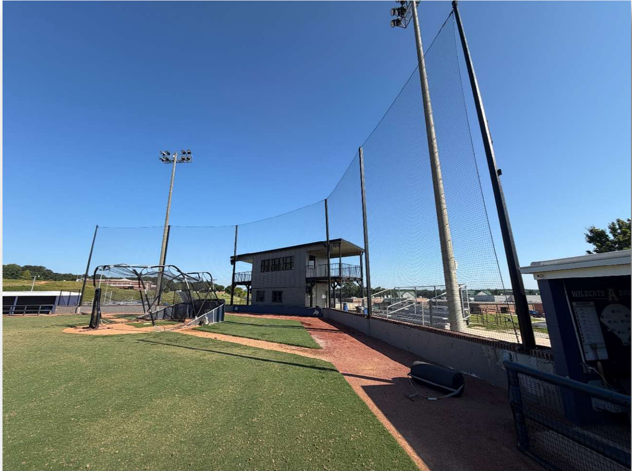
New backstop netting installed at Apalachee HS baseball field
