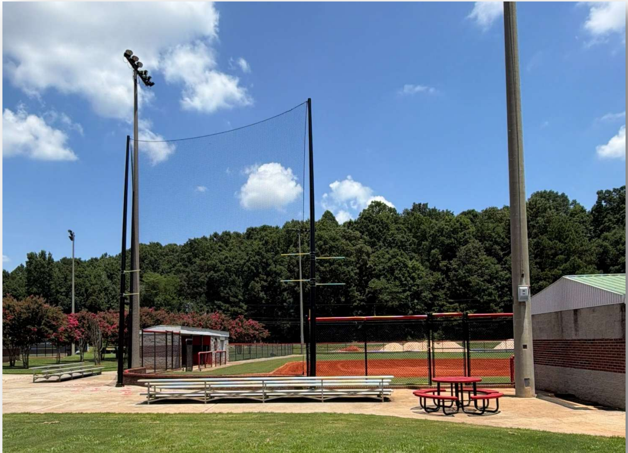
New backstop netting installed at WBHS softball field
