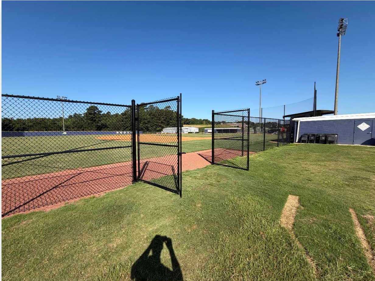
New fencing & gates installed at Apalachee HS baseball field
