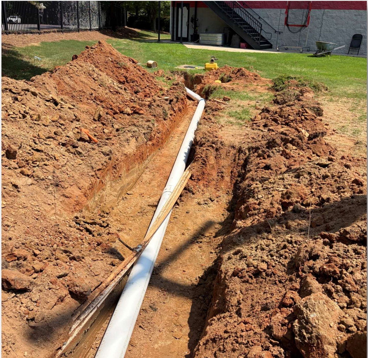
Storm drain installation at WBHS football field complete
