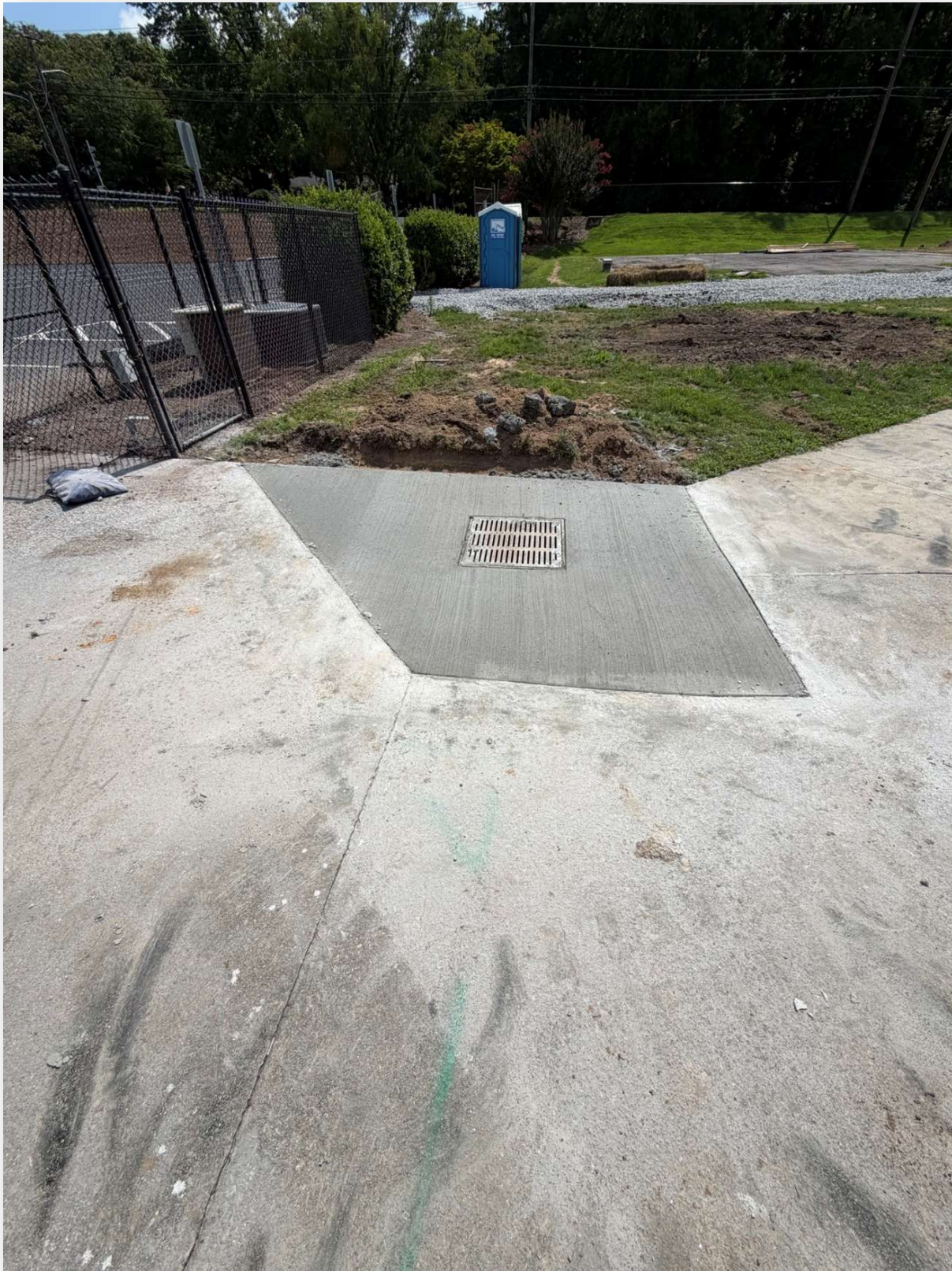
New storm drain grates installed at Winder-Barrow HS track
