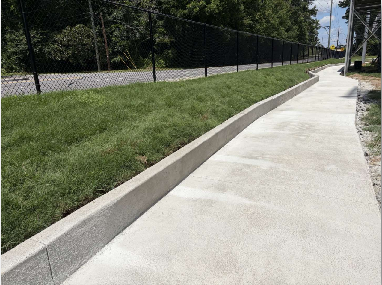
New concrete sidewalk behind Winder-Barrow HS home bleachers cont.
