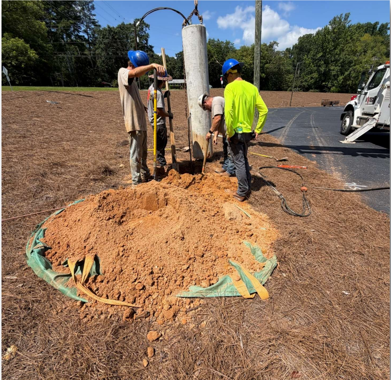
GA Power setting bases at Winder-Barrow HS parking lot
