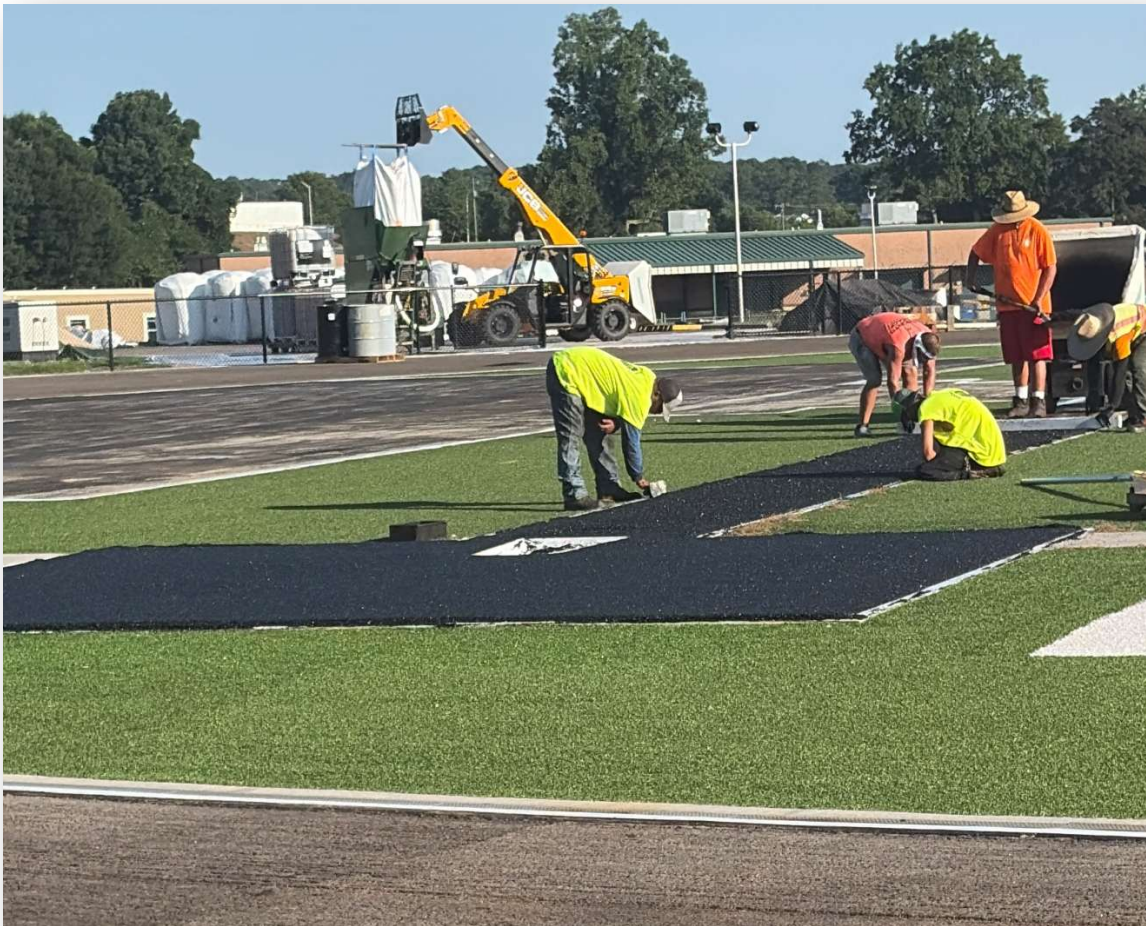
Apalachee HS track topping on-going
