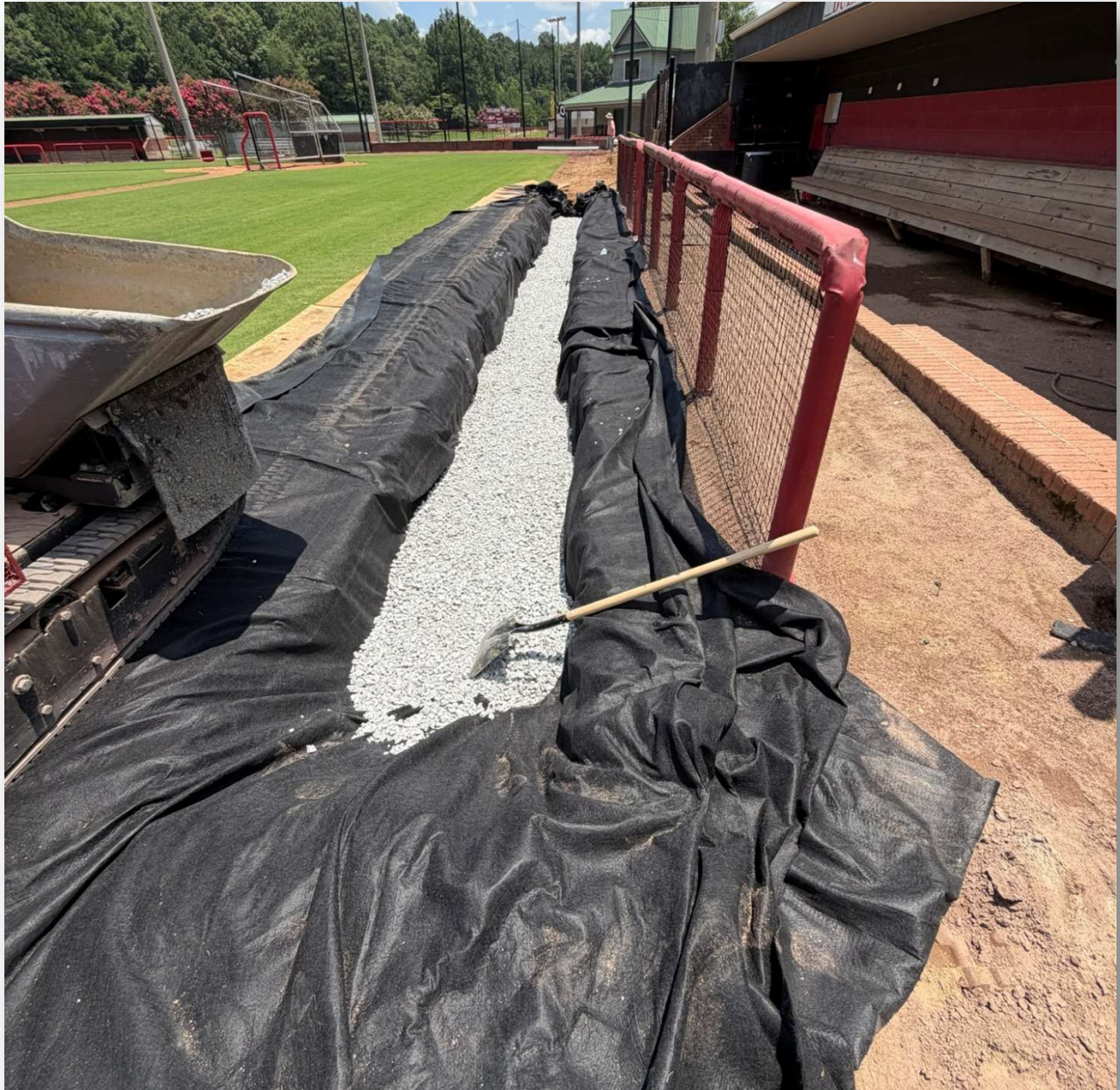
WBHS baseball maintenance drain installation on-going cont.
