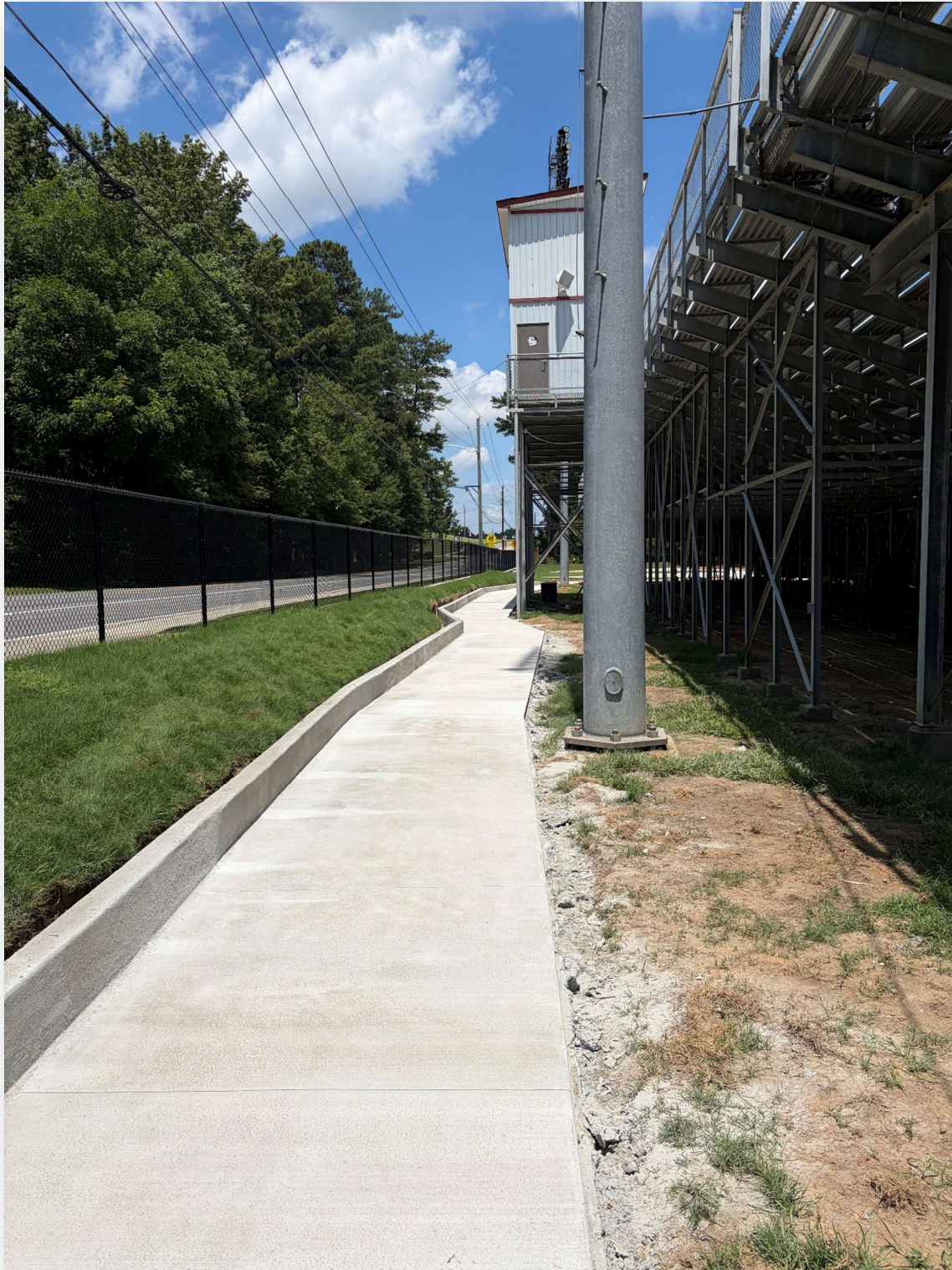
New concrete sidewalk behind Winder-Barrow HS home bleachers
