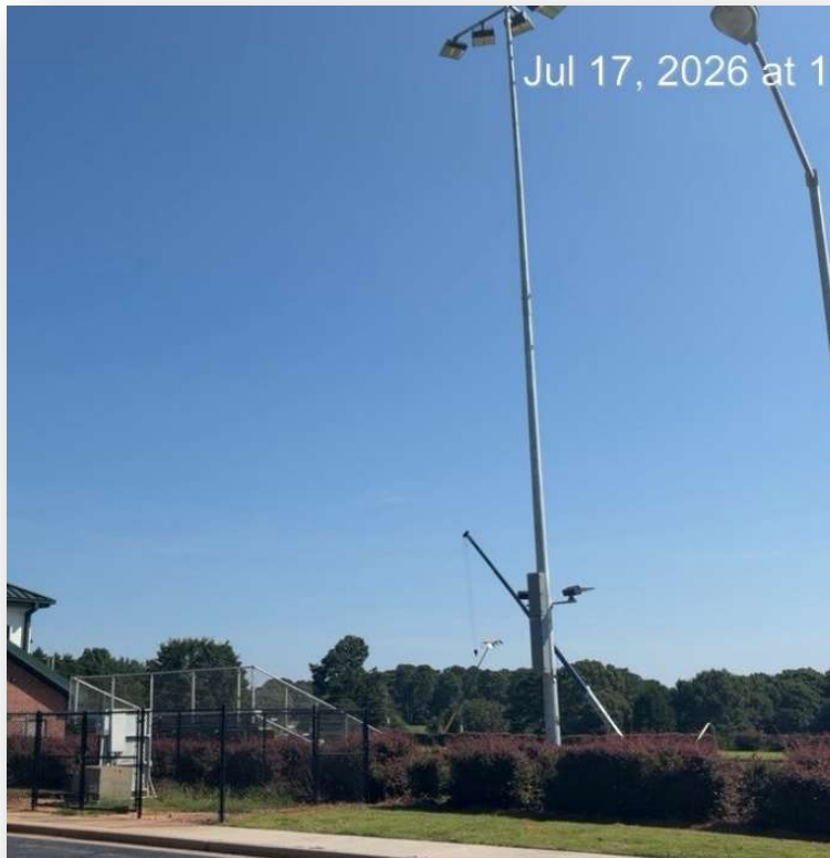
Athletic Site lighting pole installation on-going
