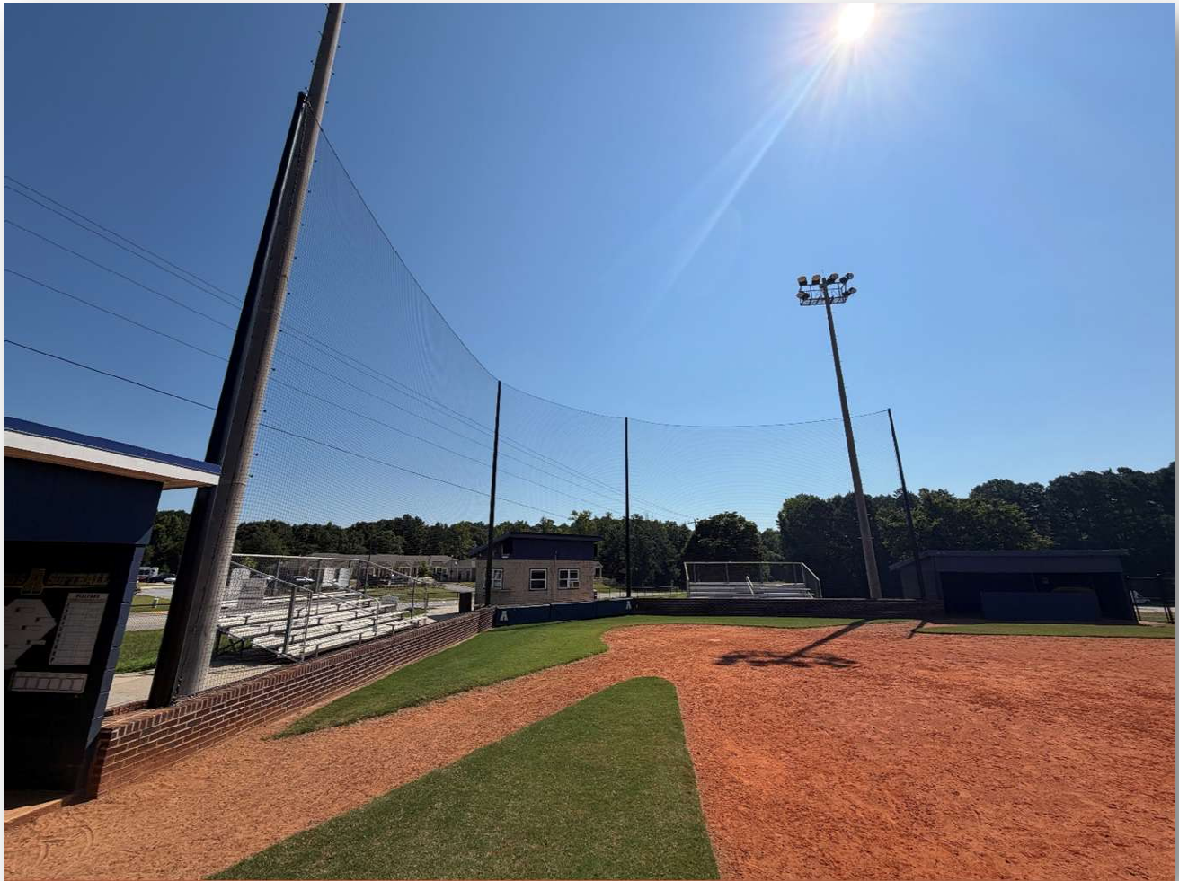
New backstop netting installed at Apalachee HS softball field
