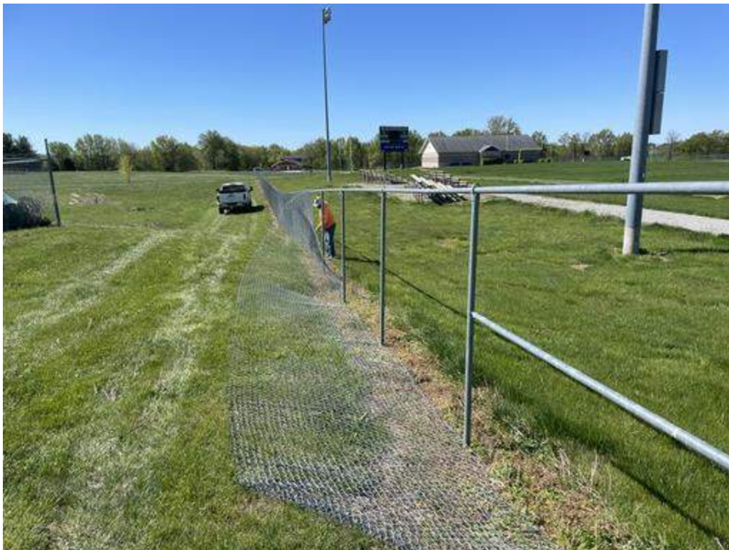
Track & Field Fence Removal - 5/2
