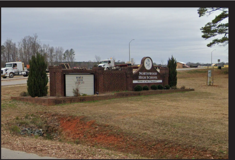
EXISTING MONUMENT: PARTIAL DEMO OF UPRIGHT FEATURES, LEAVING EXISTING PLANTER BED FOR NEW KNEE WALL AND SIGN CONSTRUCTION
