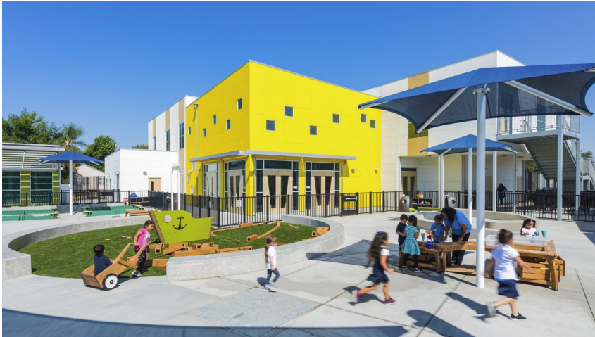
Barton Elementary School: Early Childhood Center
