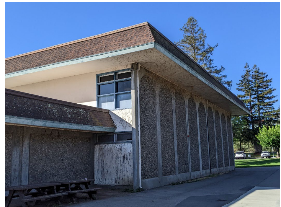
Fig. 1. Tilt-up building system.
