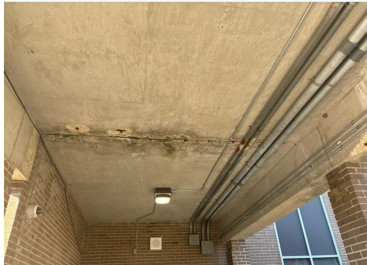
Building Envelope – John T Hoggard HS
