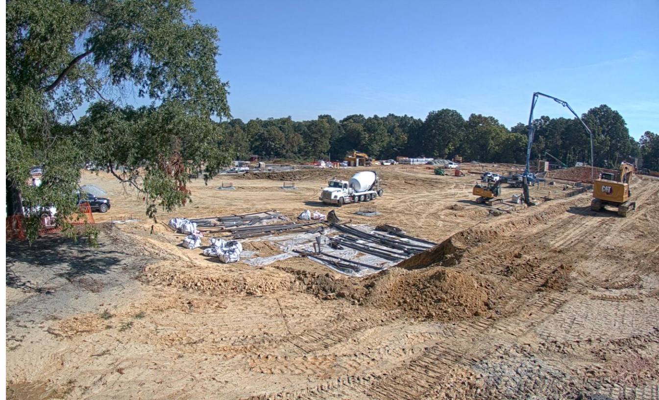
Footing installation preparation
