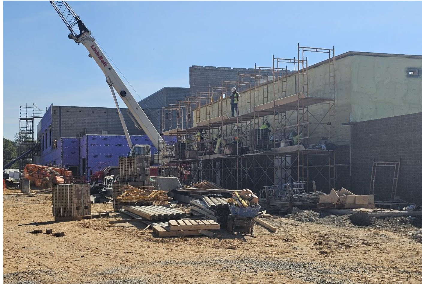
Brick Veneer Installation
