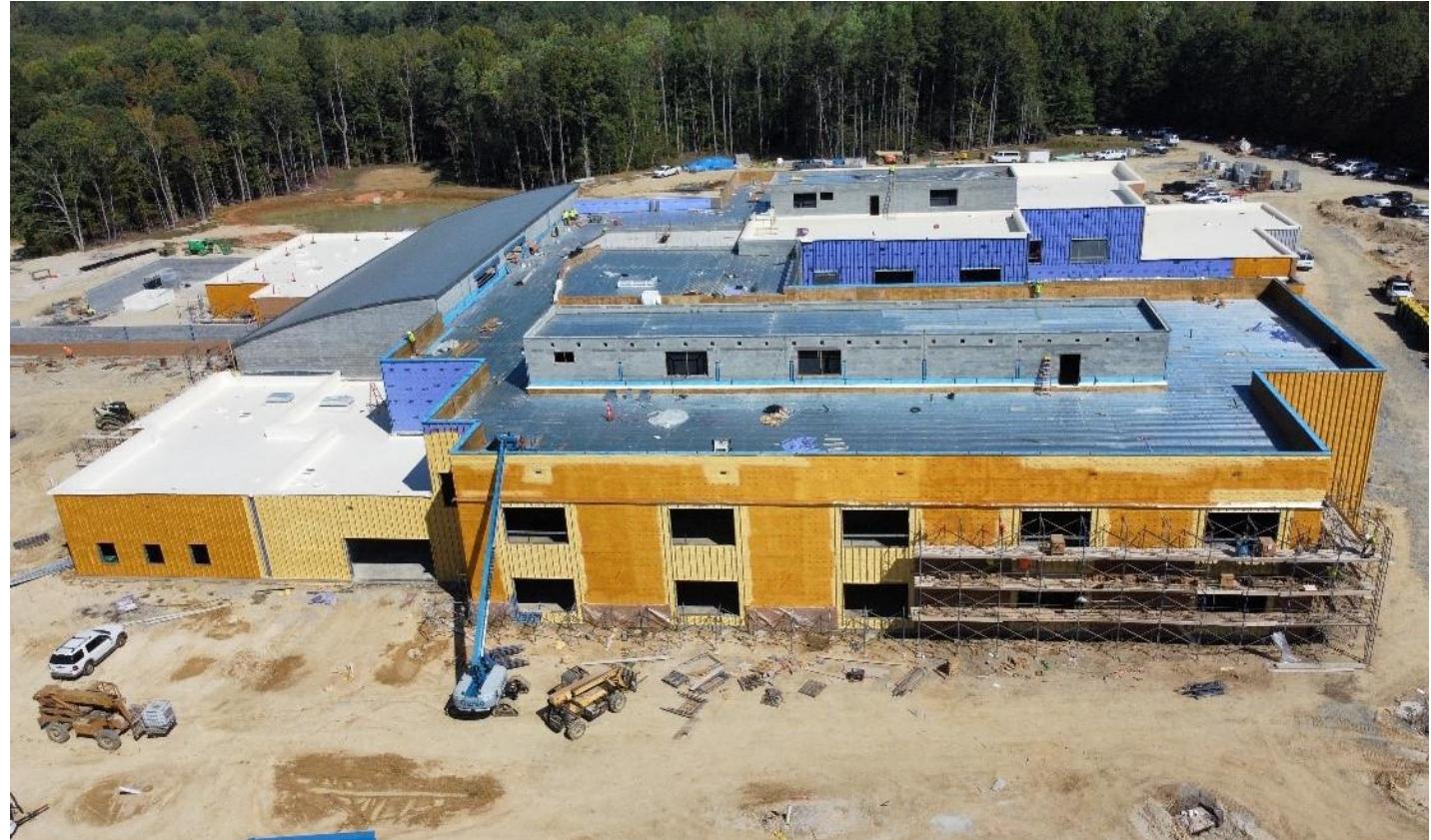
Roof and Veneer Preparation
