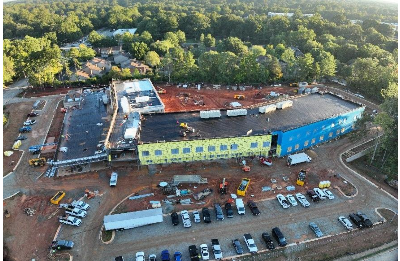
Roof and Veneer Preparation
