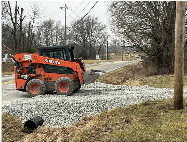
Temporary Construction Entrance
