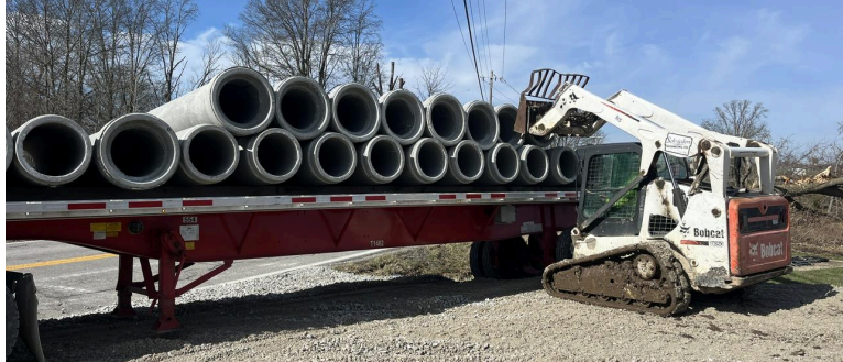
Storm Drainage Pipe Delivery
