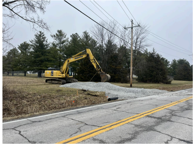
Temporary Construction Entrance
