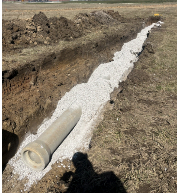
Storm Line Between Structures 7 & 8
