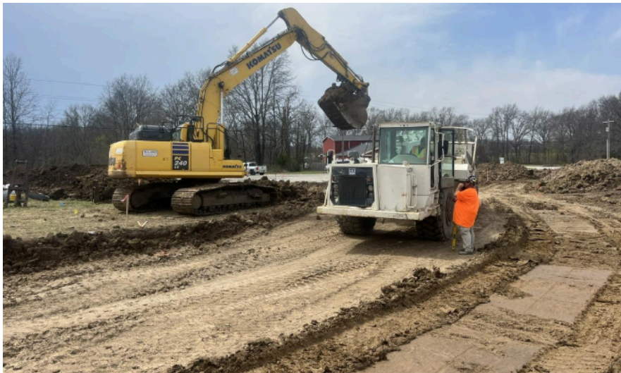
Placing Fill at Entrance Drive Lane
