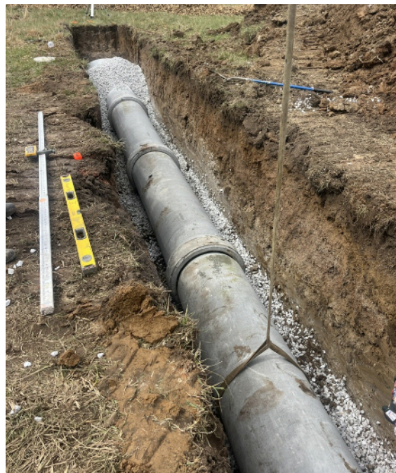
Storm Line Between Structures 5 & 6
