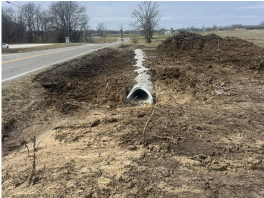
Storm Pipe & Structures 12 & 13 and Grading at Entrance
