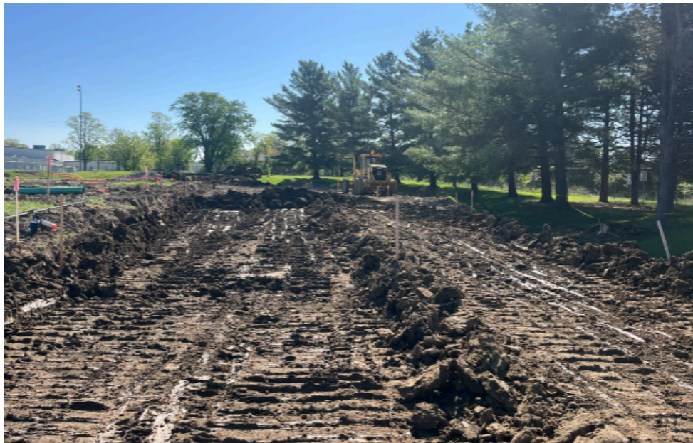
Beginning to Grade the Drive Lane
