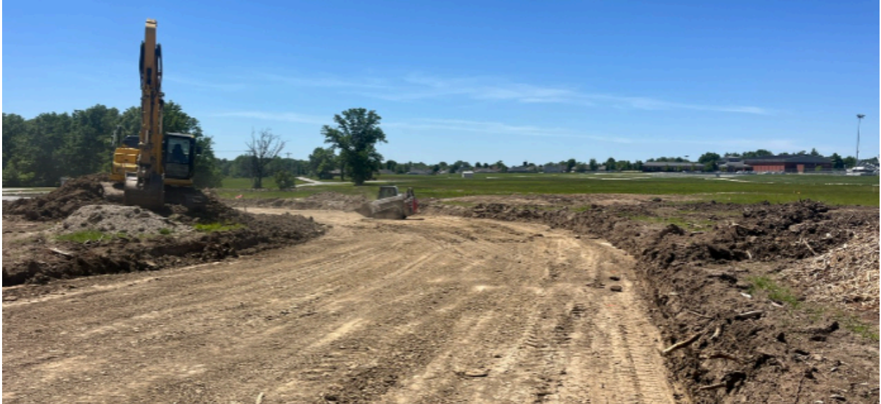
Fine Grading at the Drive Lane
