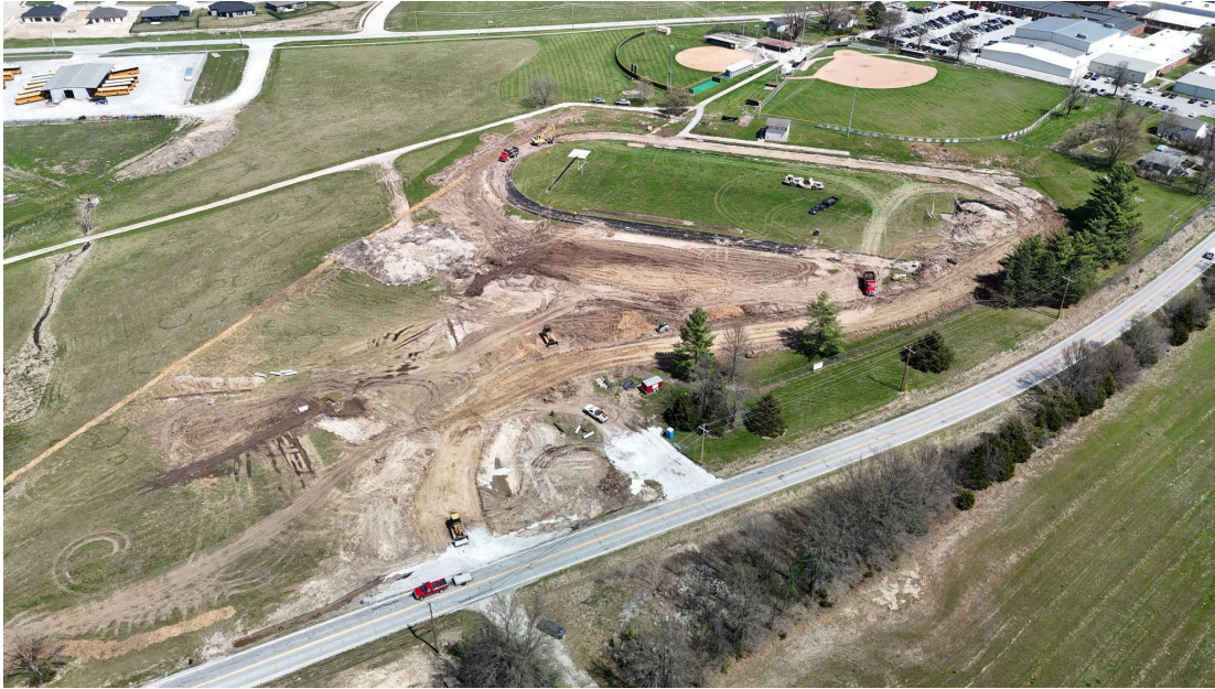
Aerial Photo of Site on April 9, 2026
