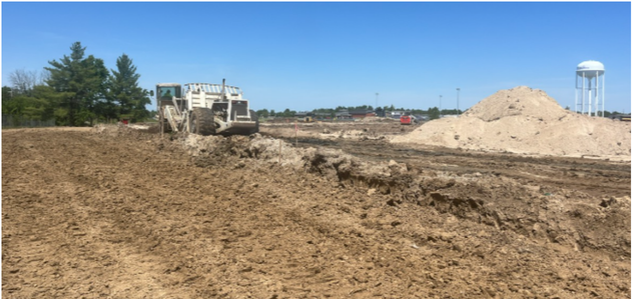
Grading at the Field
