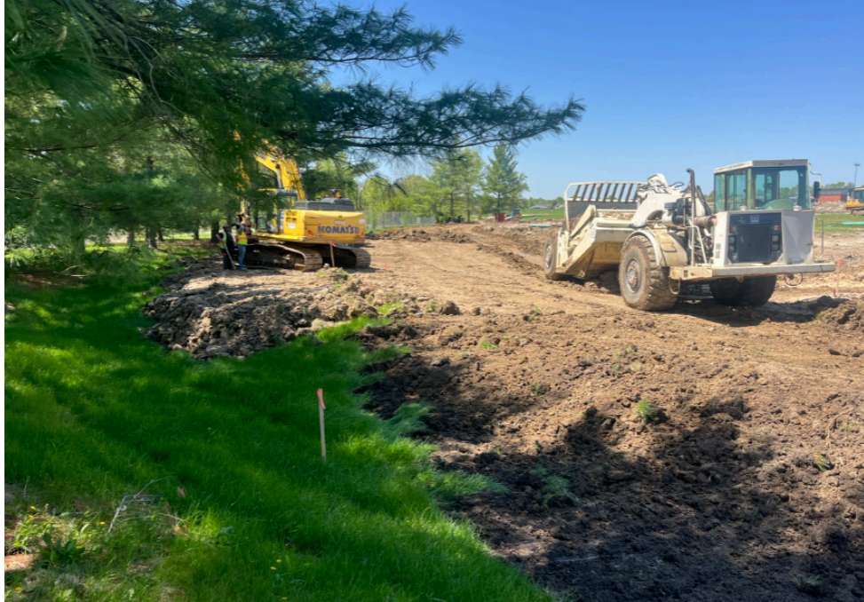
Stripping Topsoil at the Drive Lane
