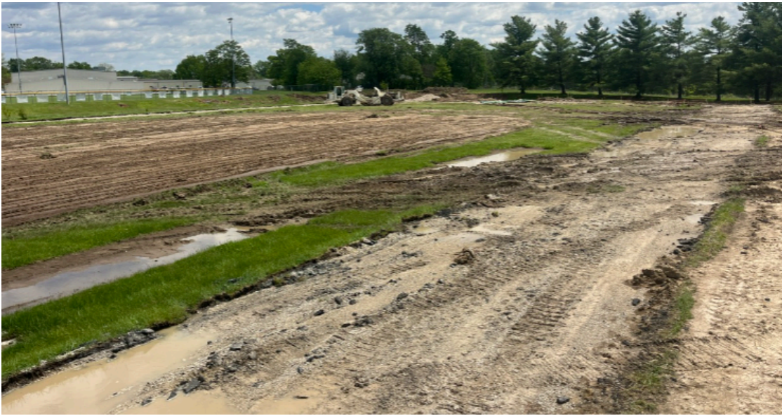
Stripping Topsoil at the Field
