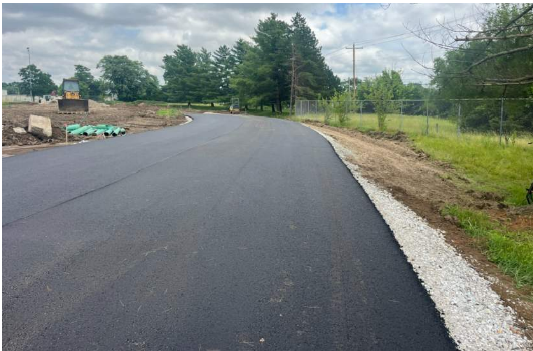
Base Course at Drive Lane
