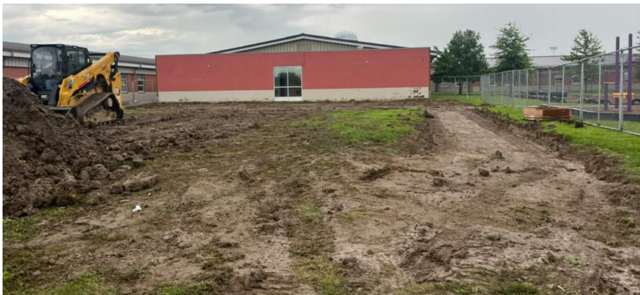
Grading at Classroom Addition
