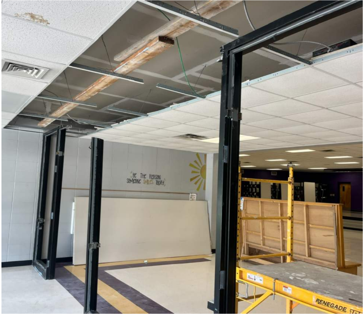
Removing Storefront at Intermediate School Main Entrance
