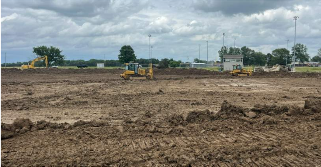
Grading at New Field
