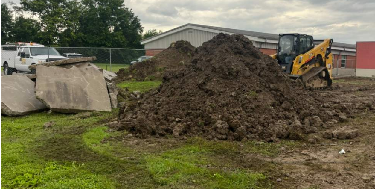
Demo at Classroom Addition
