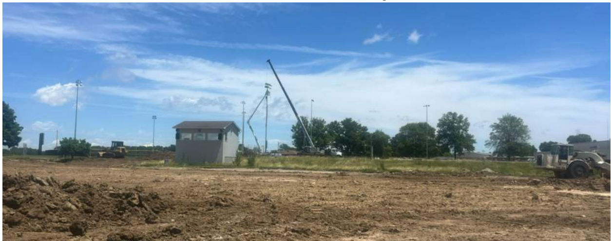
Removing Existing Field Lights
