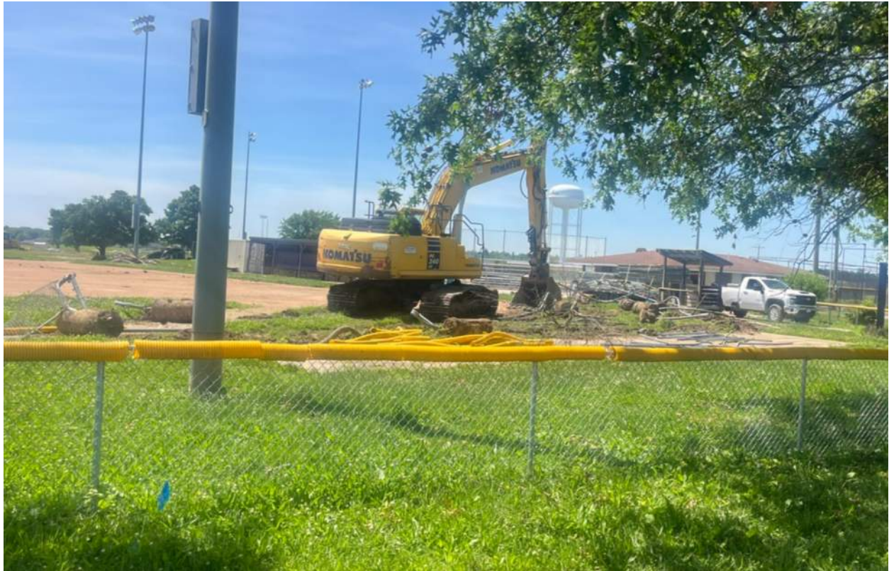
Demo at Old Field / New Parking Lot
