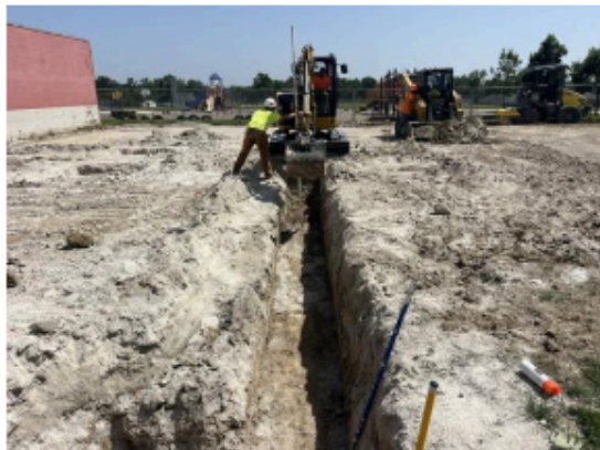
Digging footing at the addition
