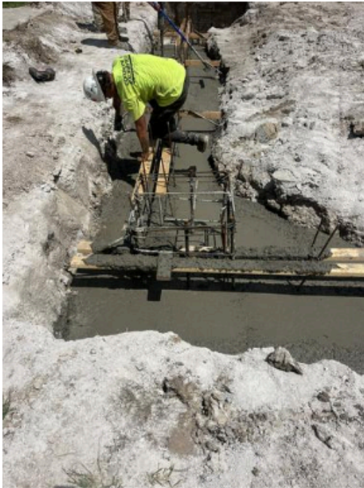
Footing at addition
