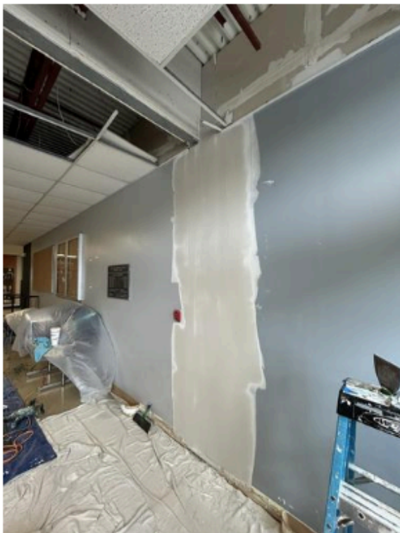
Mud and Tape at North Parking Lot
