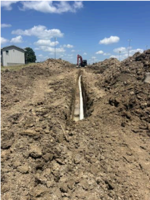
Water line work
