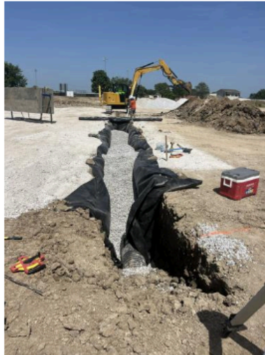
60' of storm piping
