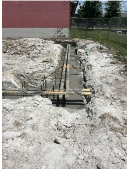
Footing at addition
