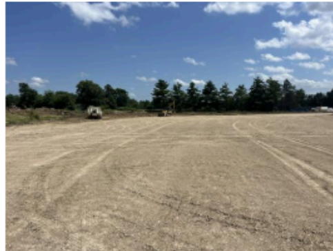
Grading on the south of the playing field
