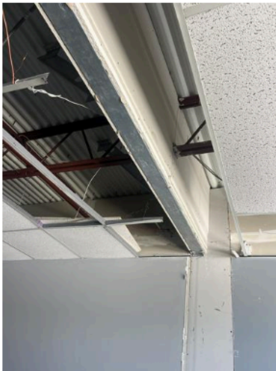
New header with drywall
