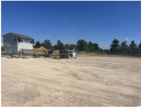
Digging out for storm work
