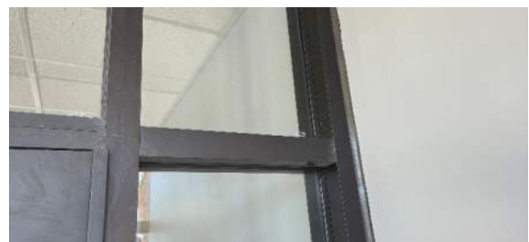
General Construction Debris Cleanup
