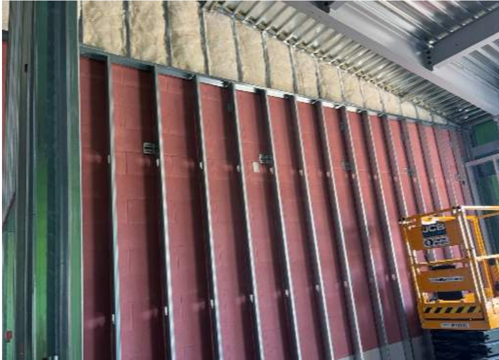
Interior Framing and Insulation
