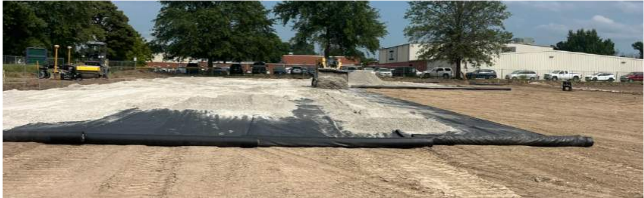
Parking Lot Rock and Fabric
