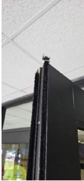
Intermediate School Entrance: Weather Stripping
