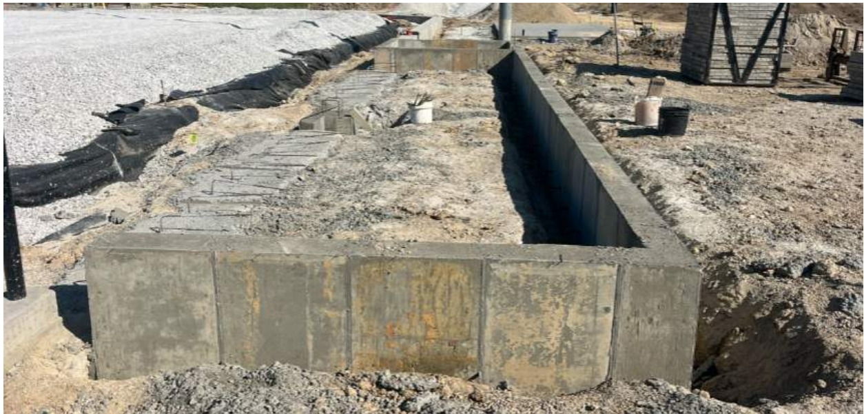
3rd Base Dugout Foundation Walls
