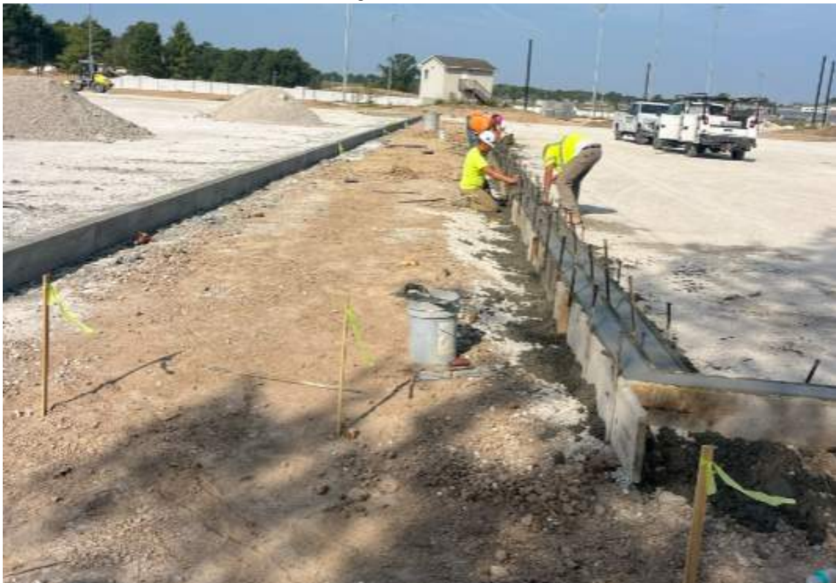
Forming & Pouring Concrete Curbs at Parking Lot
