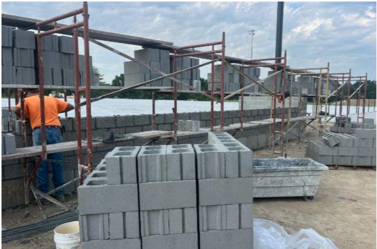
Masonry at Dugouts
