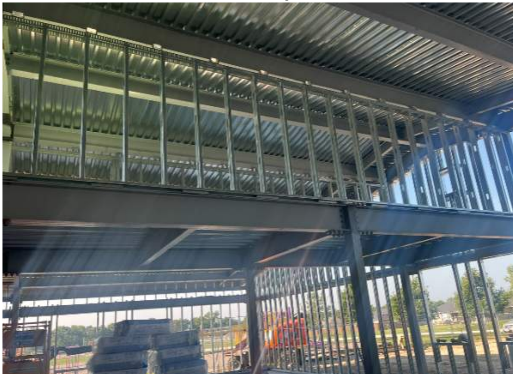
Interior Framing at the Mezzanine
