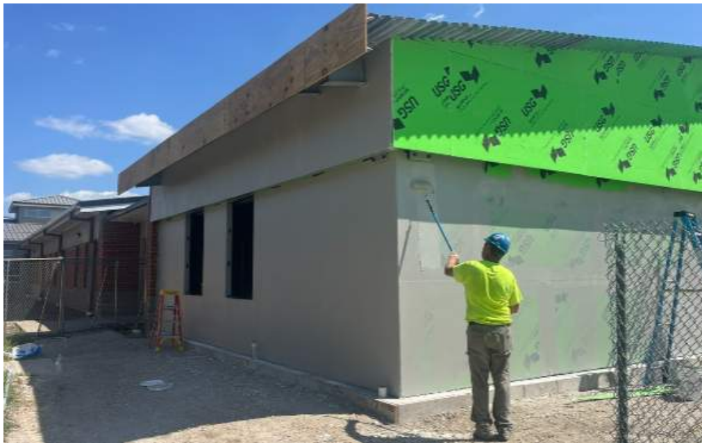
Exterior Wood Blocking & Air Barrier
