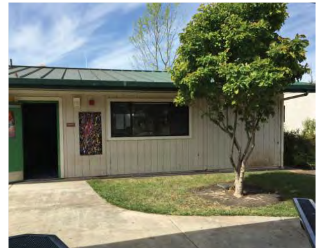
Classroom Building Exterior
