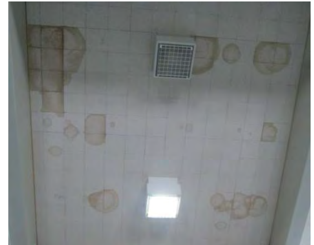
Water Damage at MPR Ceiling
