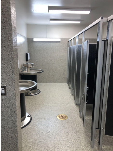
Piner HS Restroom Remodel
