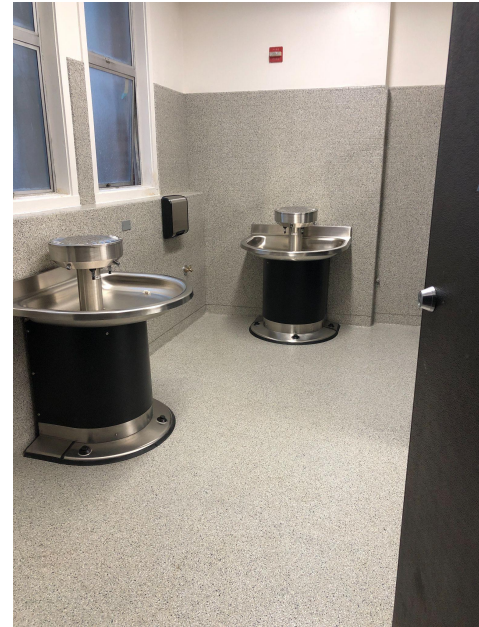
Santa Rosa HS Restroom Remodel
