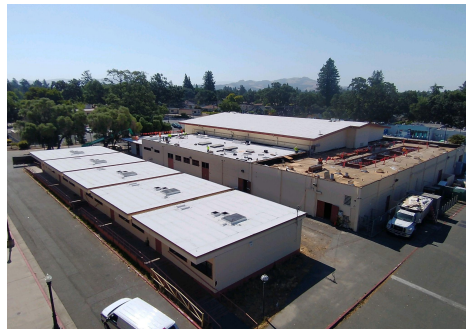
Santa Rosa HS Roofing & HVAC
