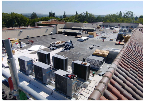
Santa Rosa HS Roofing & HVAC
