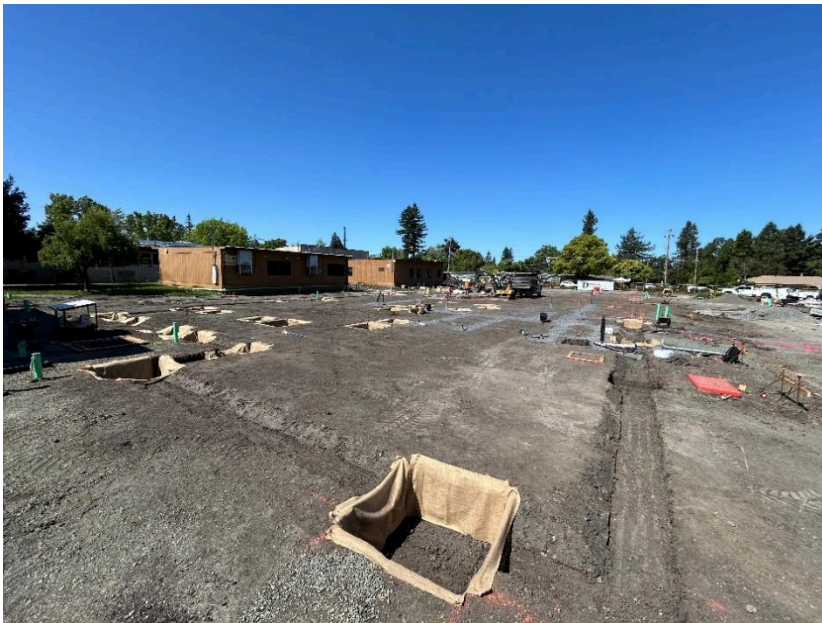
Montgomery HS Construction Site, 5/7/24
