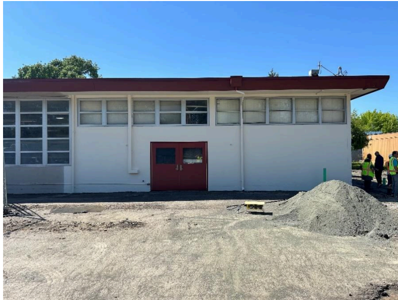
Montgomery HS Exterior Paint Mockup, 5/08/24
