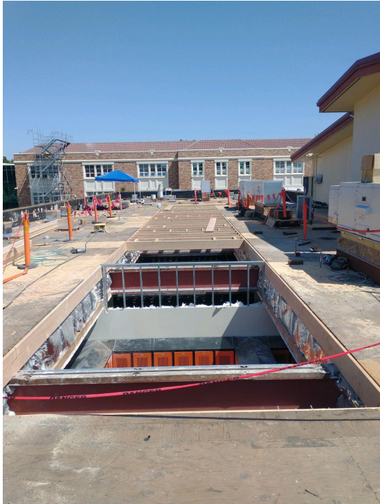
Santa Rosa HS Roofing & HVAC
