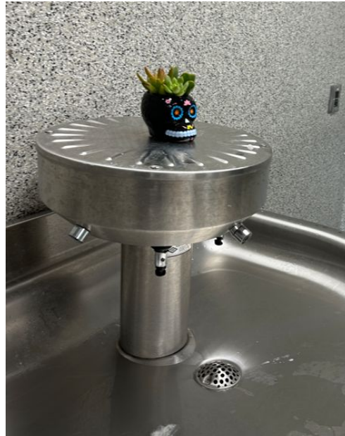
Ridgway HS Restroom Remodel
