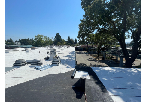
CCLA Roofing & HVAC
